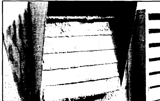
Figure 3. Dust on an air vent from a Chicken Barn.
