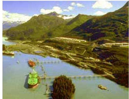
Aerial photo of the Valdez Marine Terminal, where crude oil is loaded from the Trans-Alaska pipeline onto tankers for shipment to markets. It was here that oil was loaded onto the Exxon Valdez for shipment to Los Angeles. Click image for larger view and further details.
