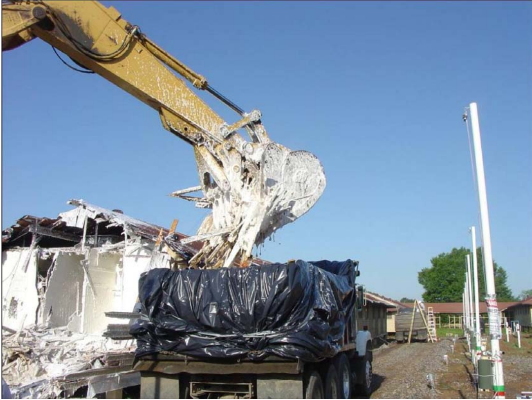
Figure 4-33. Loading the AACM demolition debris.
