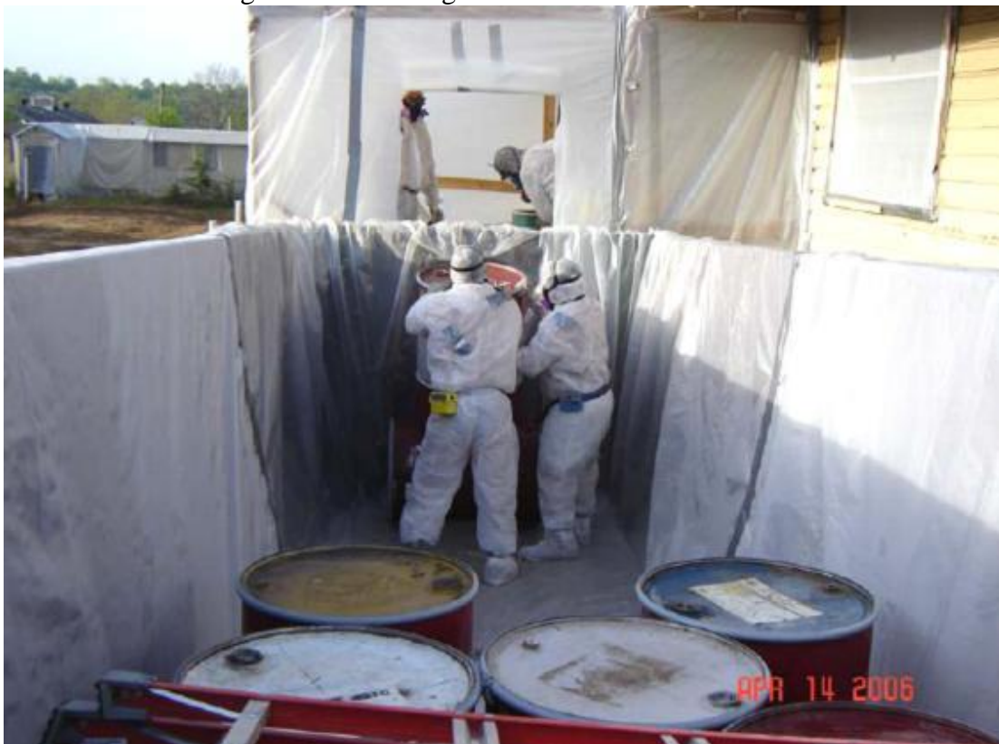
Figure 4-5. Loading asbestos-containing material into roll-off container.
