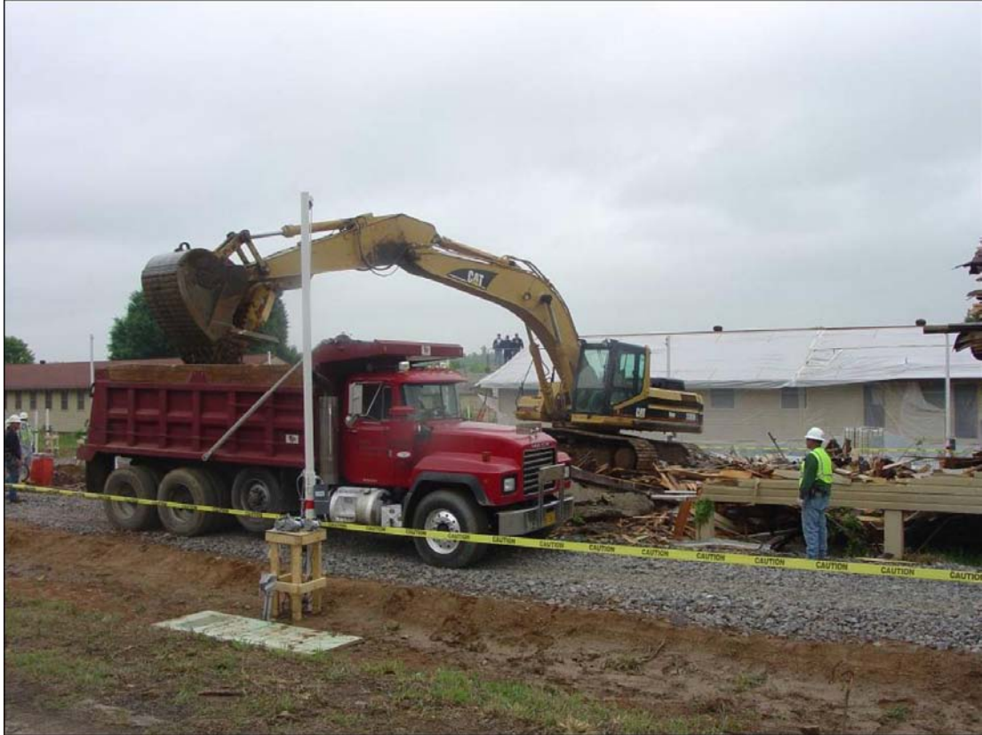
Figure 4-19. Finishing NESHAP demolition.
