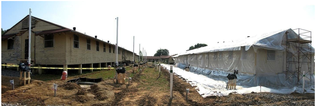
Figure 4-16. Preparation of site prior to demolition of NESHAP Method building (left).
