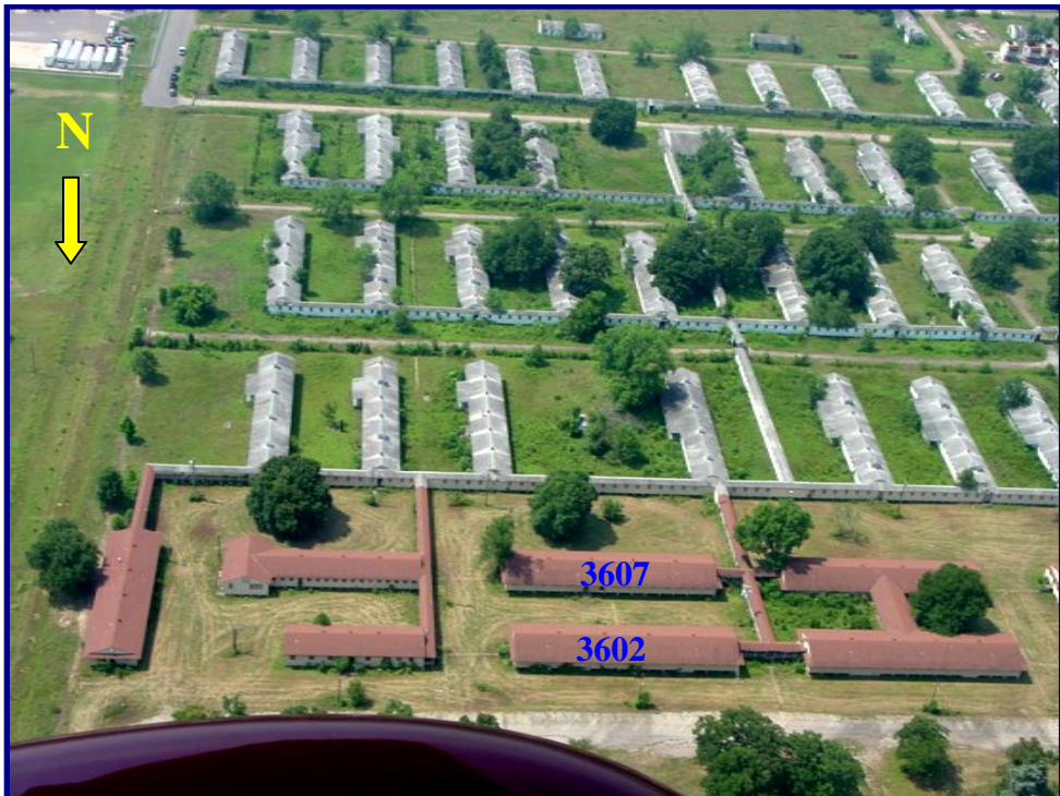
Figure 3-1. Project location at Fort Chaffee. Buildings selected for demolition are #3602 (NESHAP Method) and #3607 (AACM).
