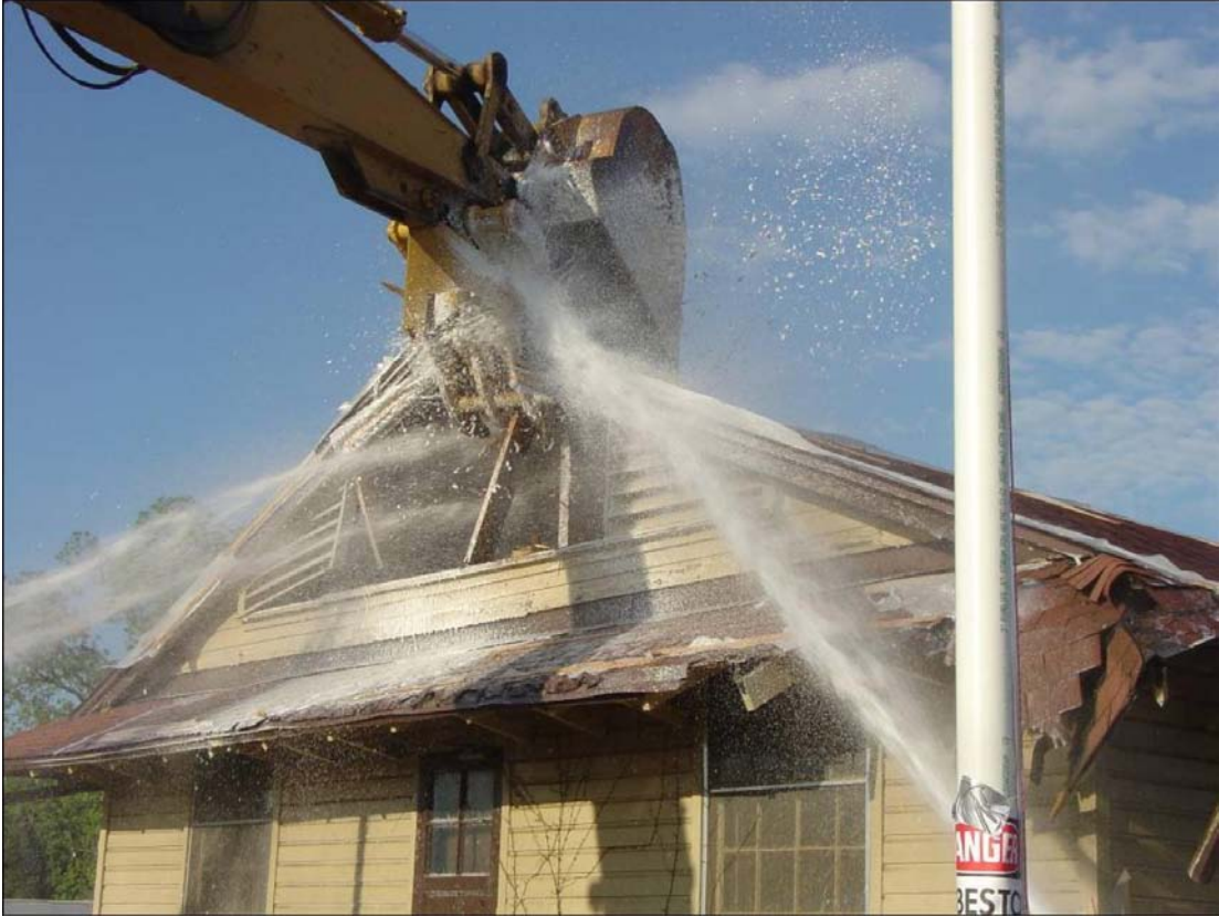
Figure 4-31. Starting the AACM demolition.
