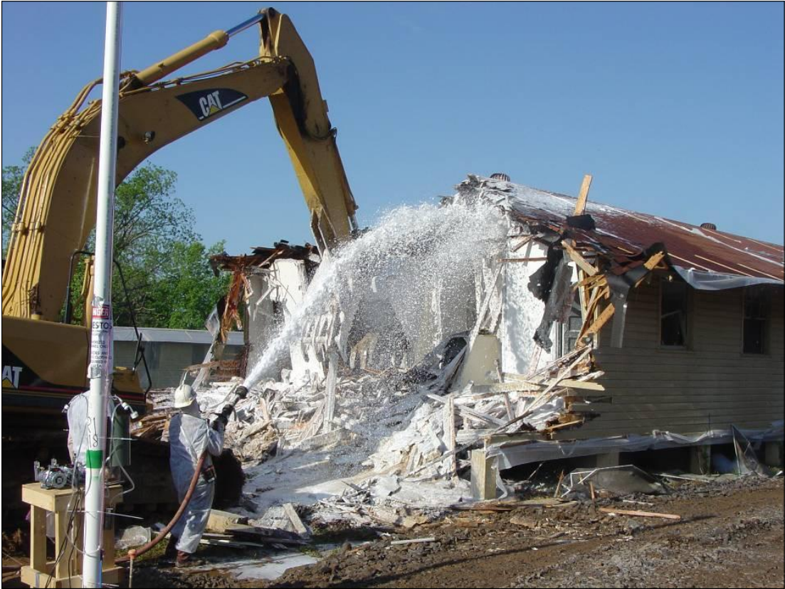
Figure 4-32. Progressing with the AACM demolition.
