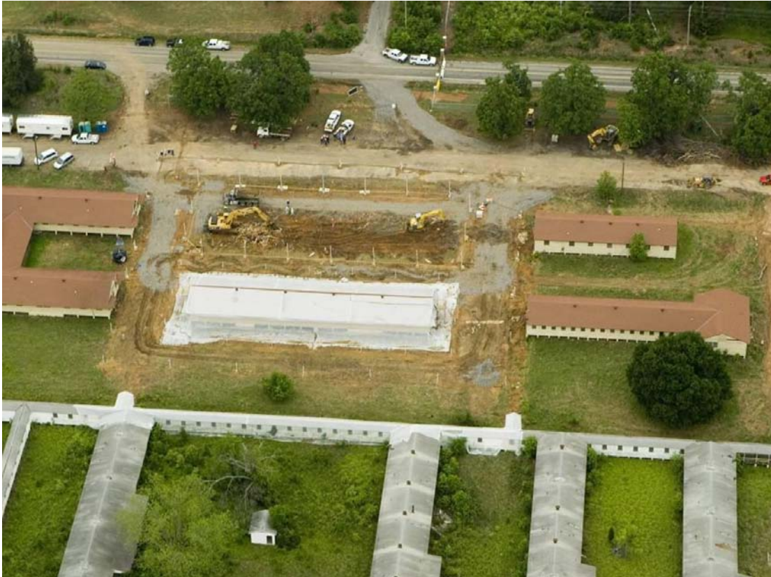
Figure 4-20. Aerial view showing NESHAP building nearly demolished.
