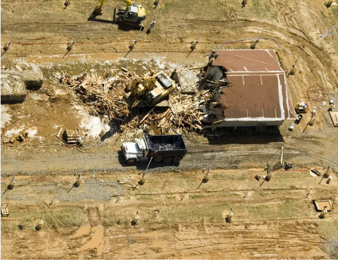
Figure 4-37. An aerial view nearing completion of the AACM demolition.
