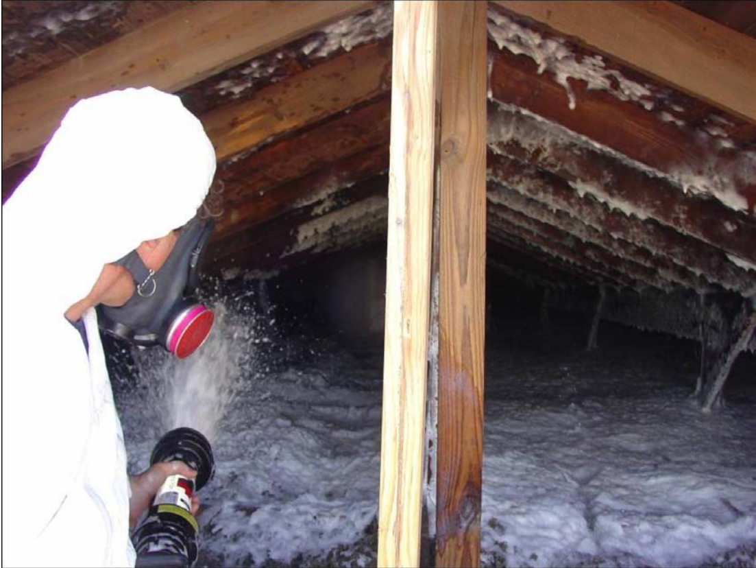
Figure 4-25. Pre-wetting the attic with Amended Water.
