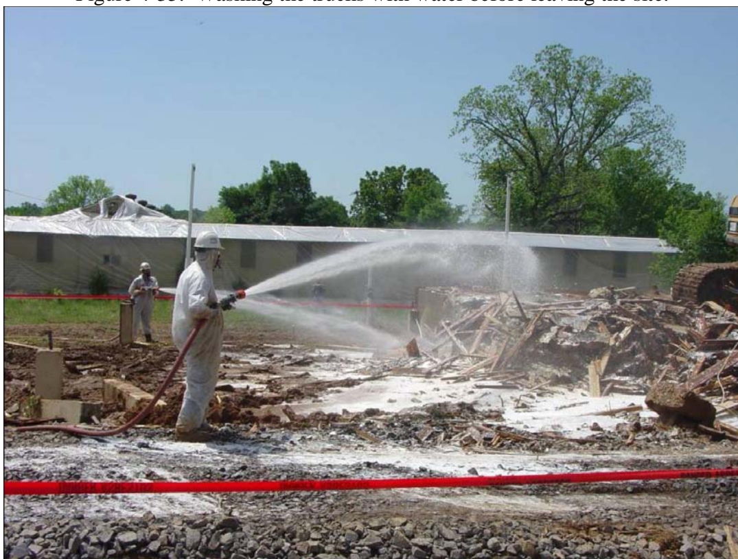
Figure 4-36. Nearing the completion of the AACM demolition.
