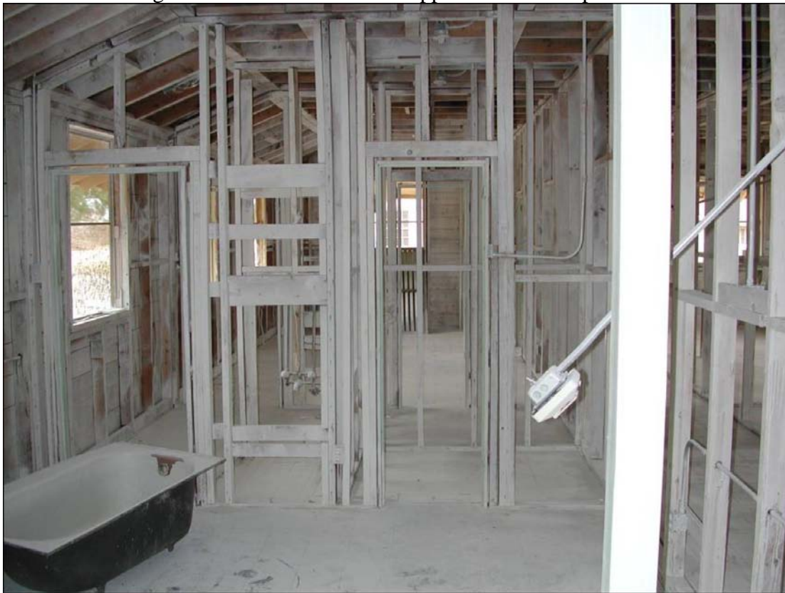
Figure 4-7. Abated area after final clearance.
