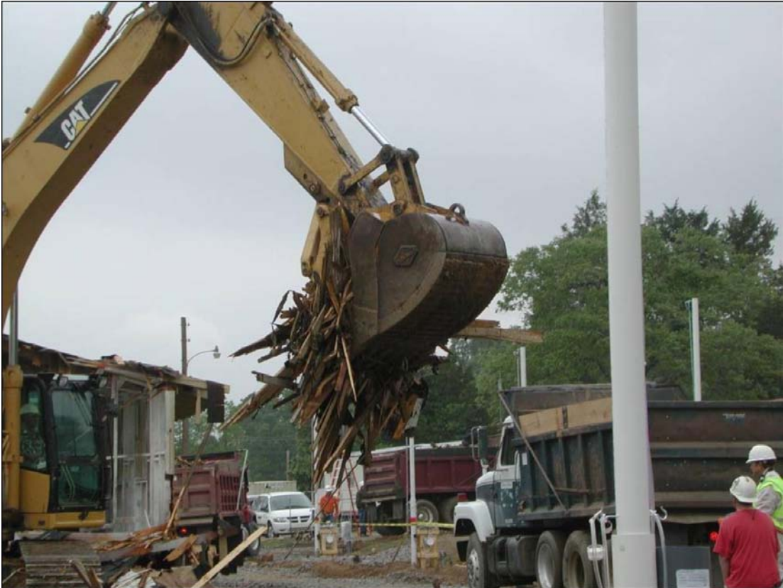
Figure 4-18. Loading NESHAP debris into trucks.
