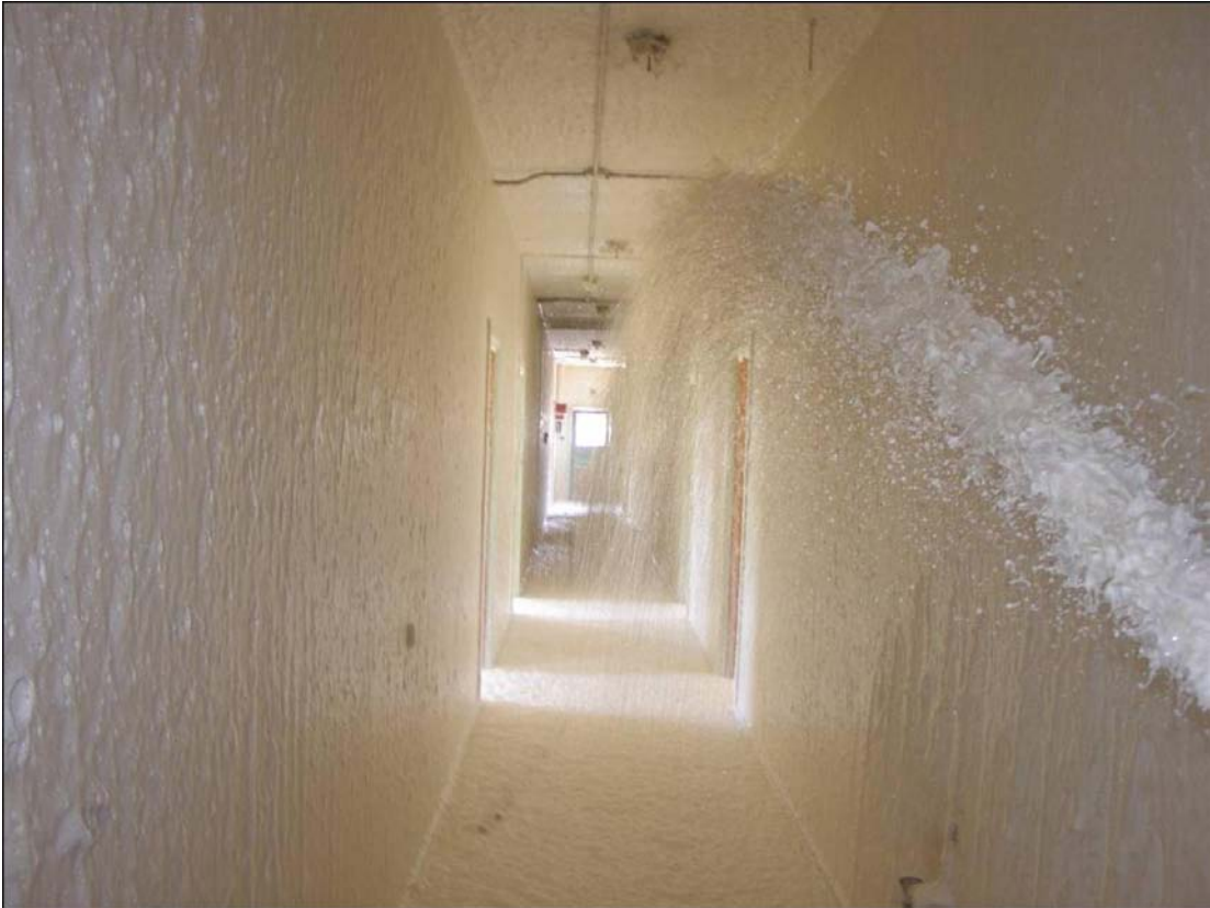
Figure 4-24. Pre-wetting the hallway with Amended Water.
