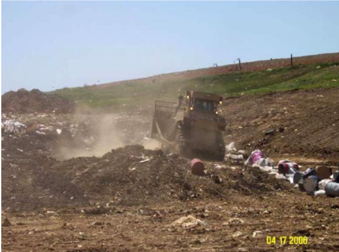
Figure 4-8. Covering abatement debris at the landfill.
