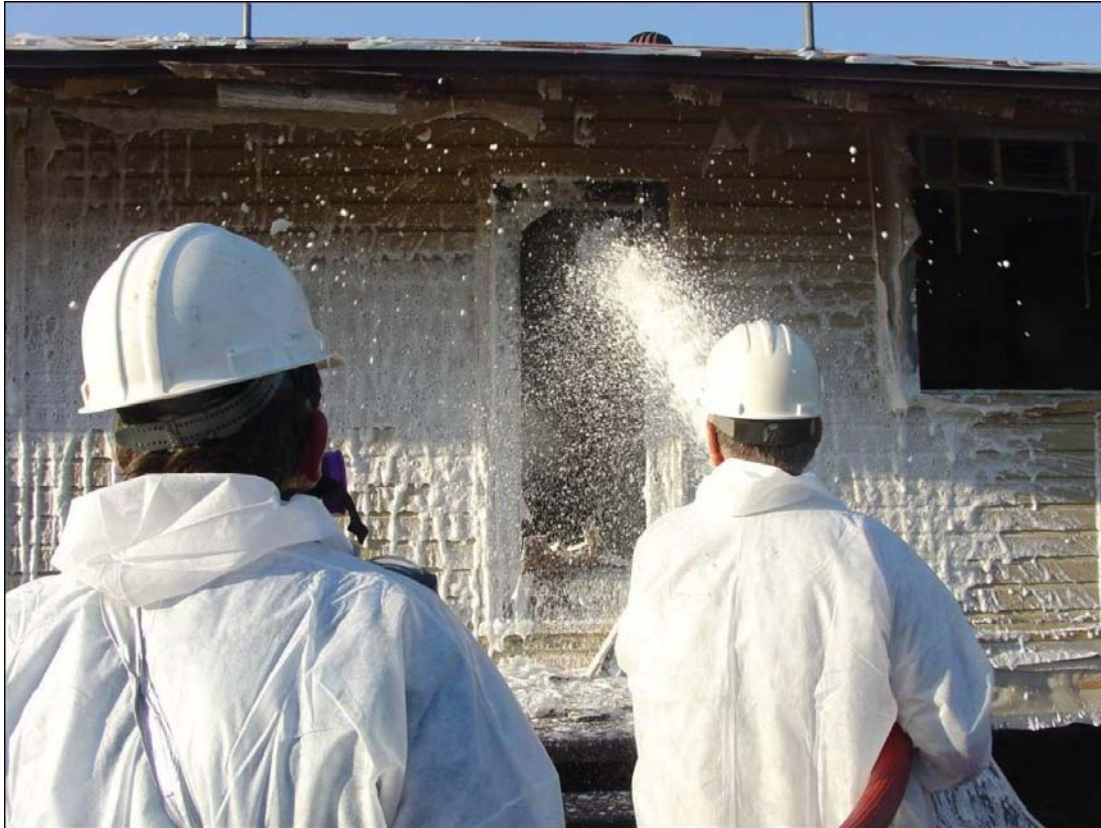
Figure 4-28. Wetting through openings on the day of the AACM demolition.
