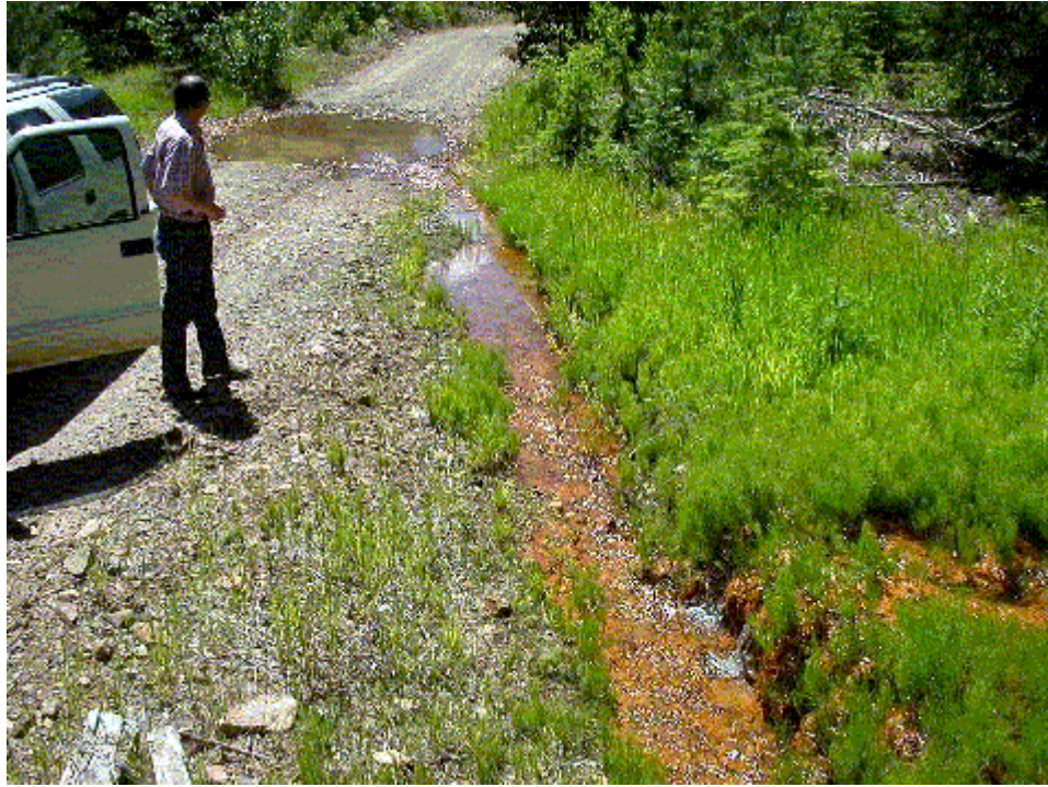
Figure 1-2. NSM site prior to technology implementation. Mine discharge shown flowing over road into Highland Creek.
