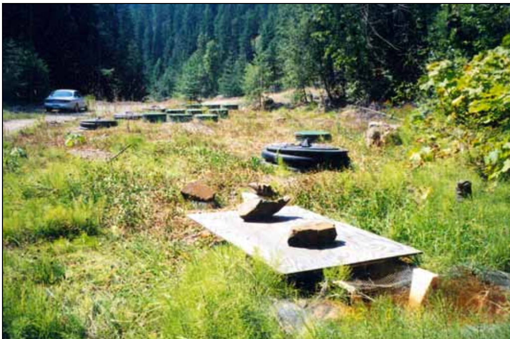
Figure 2-13. NSM ATS 2 years after installation looking downstream (September 2004).
