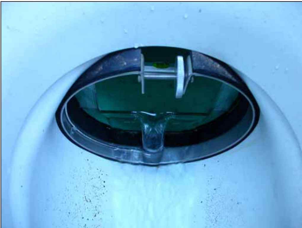
Figure 2-6. Thel-Mar weir and bubbler used to measure flow from treatment tanks.
