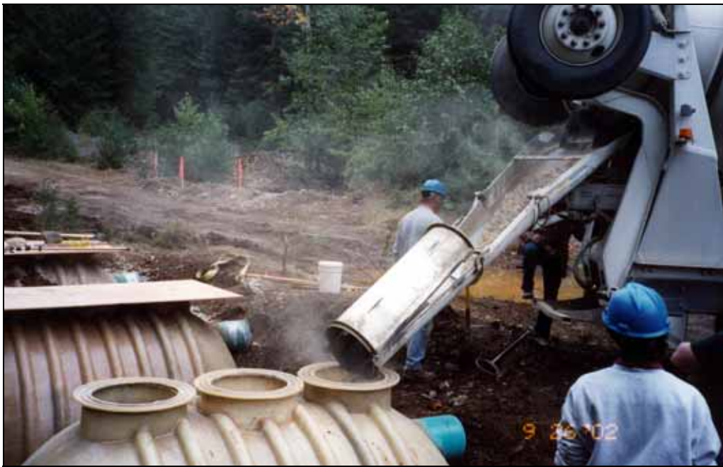
Figure 2-15. Installation of whole-bone apatite and gravel mixture into treatment tanks.
