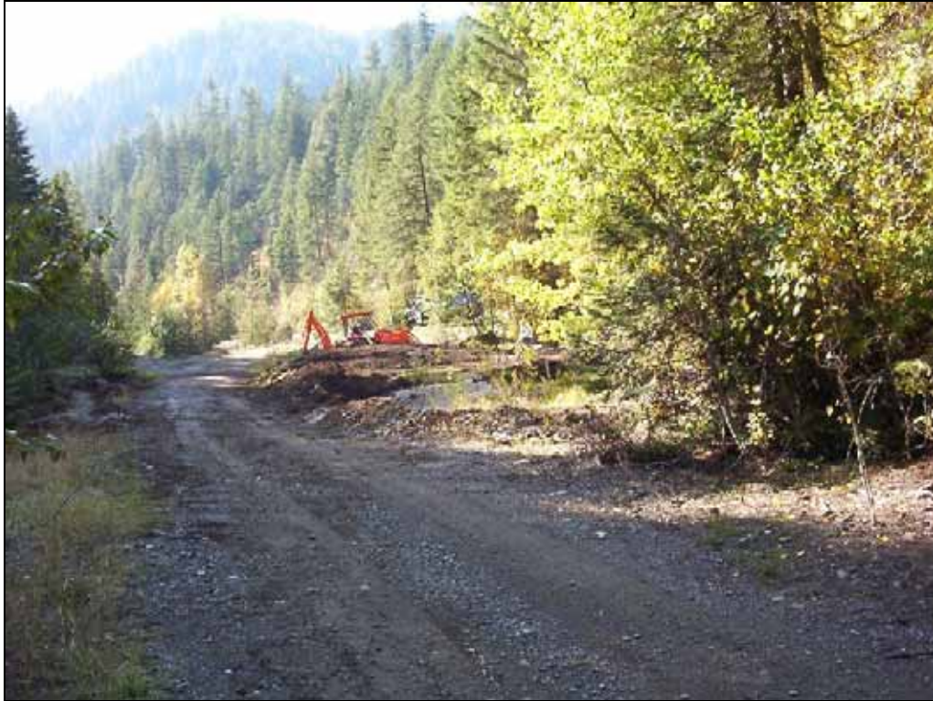
Figure 2-14. NSM ATS after closure of system.
