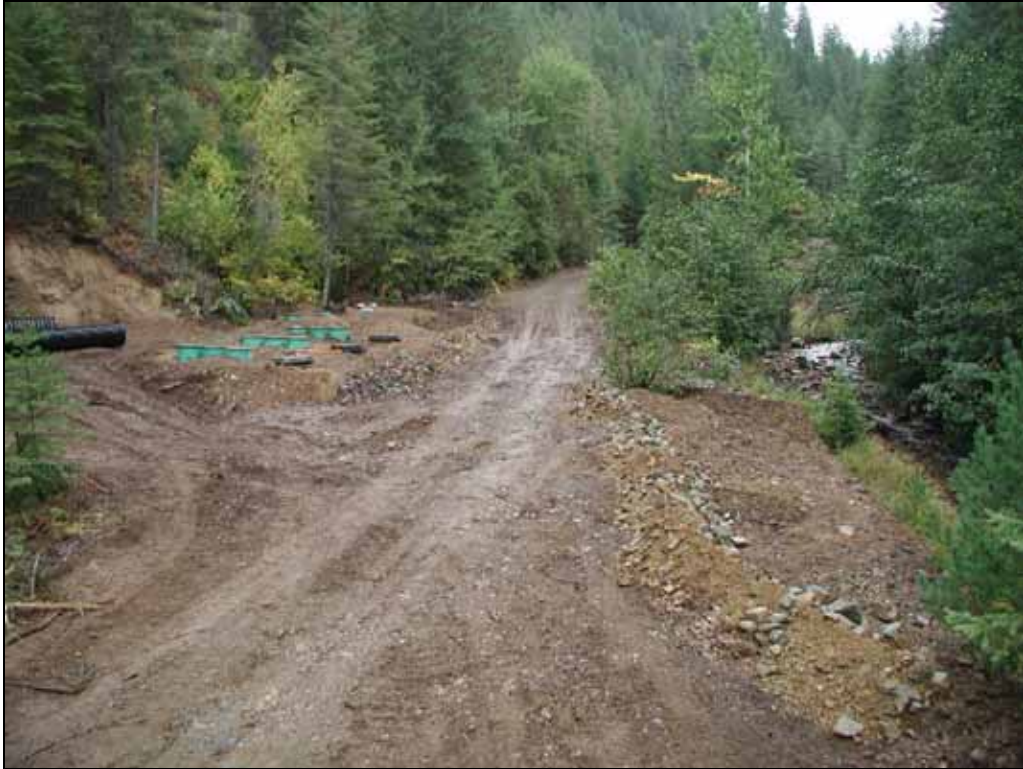
Figure 2-12. NSM ATS just after construction looking upstream (November 2002).
