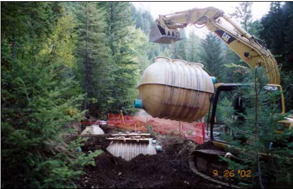
Figure 2-9. ATS Tank 4 being placed at NSM.
