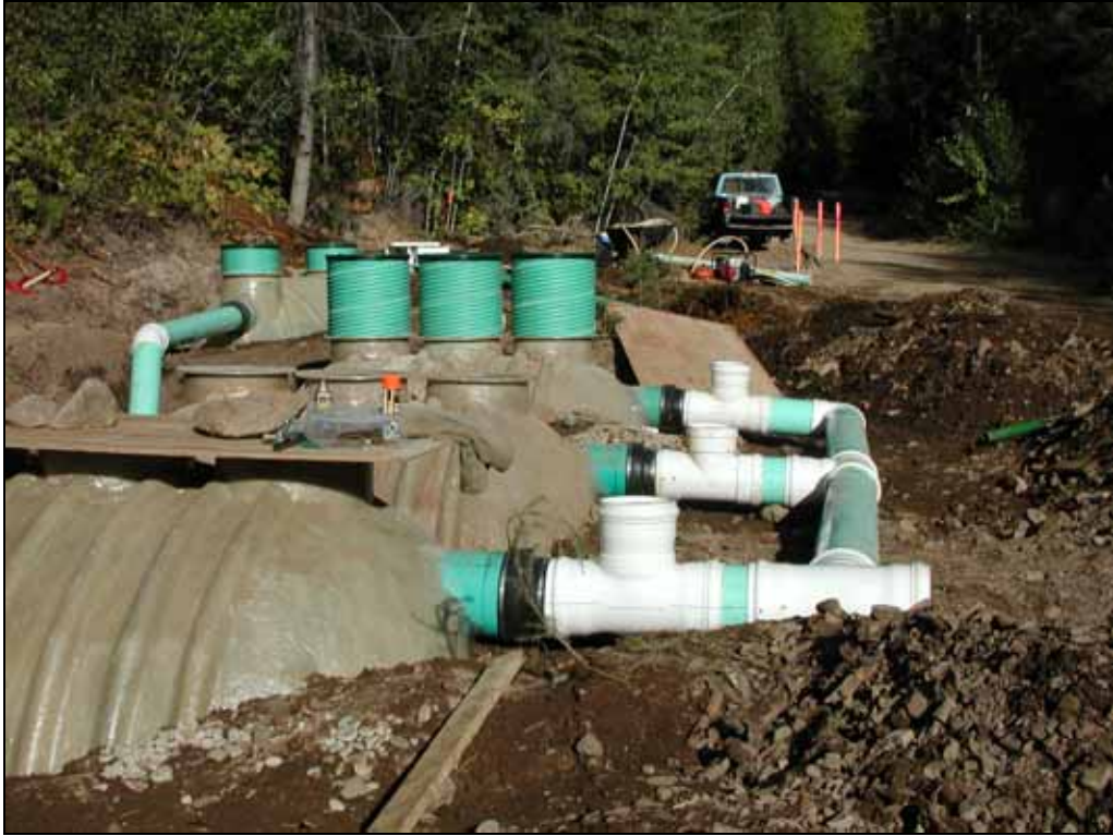
Figure 2-10. NSM ATS construction prior to covering system.
