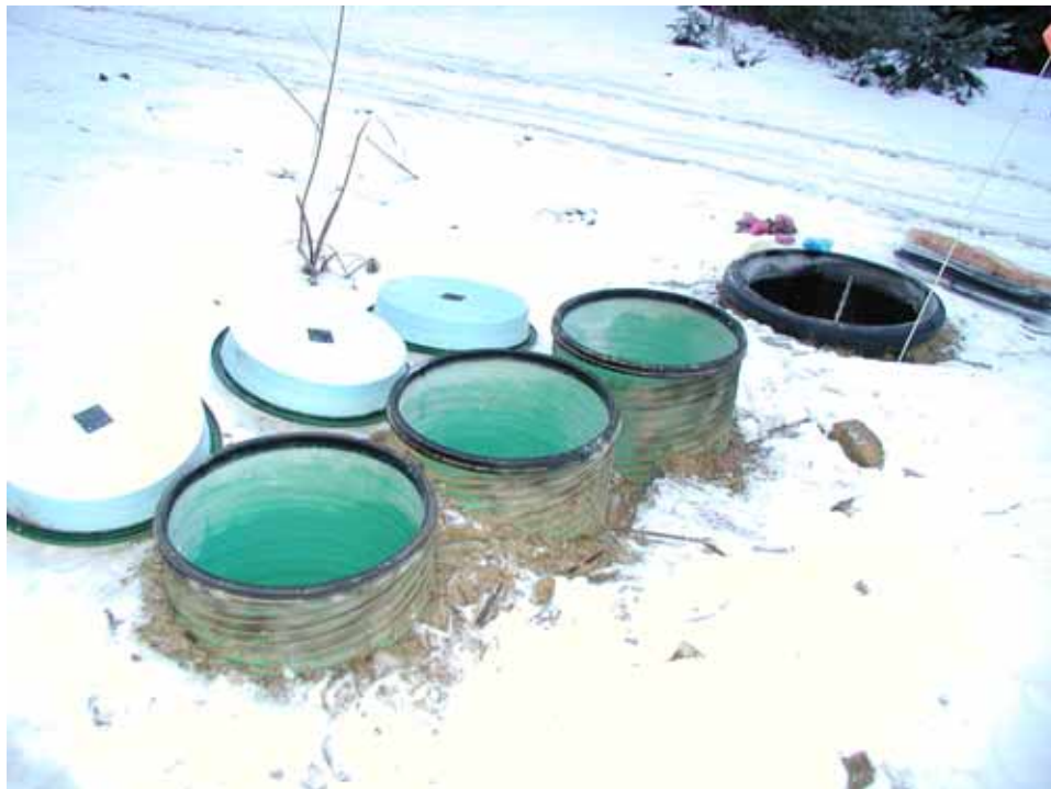
Figure 1-3. NSM site under winter conditions.
