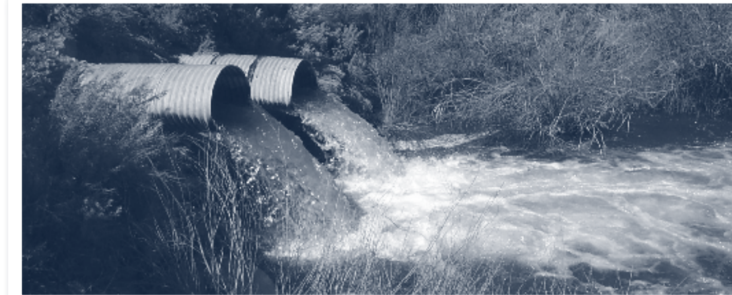
Beaver Creek during spring runoff. The height of the "waterfall" creates a barrier that prevents fish and other aquatic species from swimming upstream.
