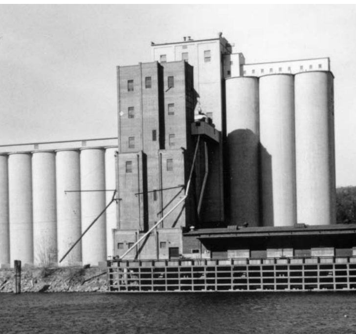
FIGURE 7. Farmers’ Union Grain Terminal Association complex, 1955. The St. Paul Municipal Grain Elevator and Sack House lie in the forefront of the complex at the right. Minnesota Historical Society.
