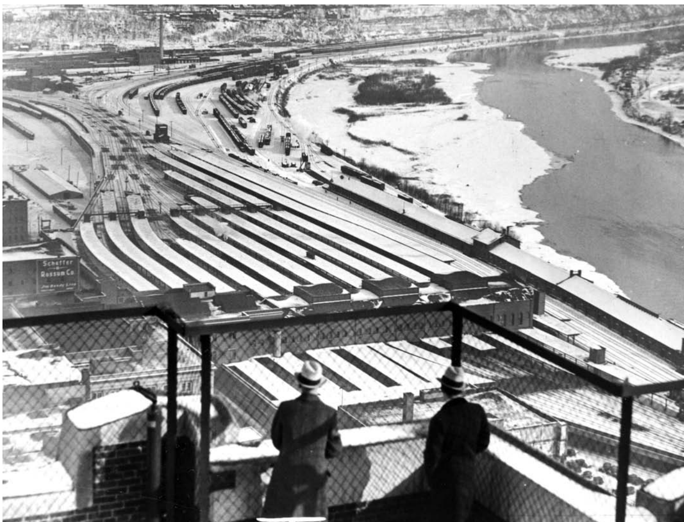
FIGURE 11. Railroads and low water undermined the Mississippi River as a commercial navigation route before locks and dams. Taken in 1931, this photograph captures the river immediately prior to the flooding of Pool 2. Photo by St. Paul Daily News. Minnesota Historical Society.
