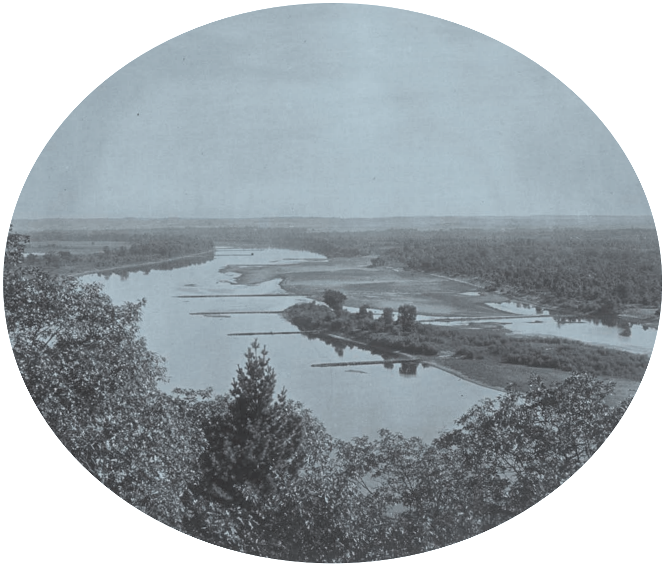
FIGURE 10. Channel constriction at Pine Bend, Minnesota, 1891. Photo by Henry P. Bosse. St. Paul District, Corps of Engineers.
