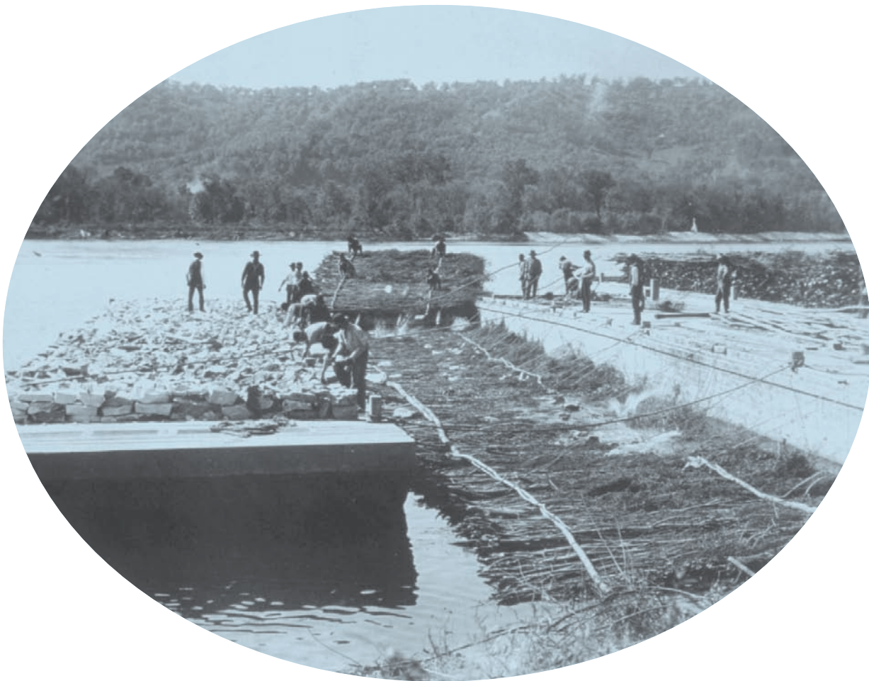
FIGURE 9. Wing dam construction. Photo by Henry P. Bosse. St. Paul District, Corps of Engineers.
