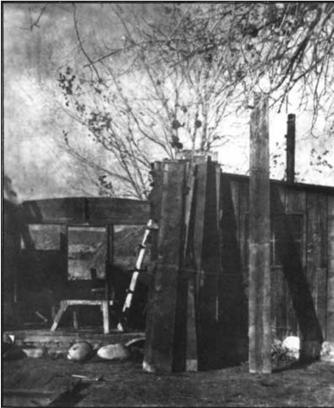
Figure 7.6. Dismantling the American Museum storage shed at rear of Morris house, 1934.
