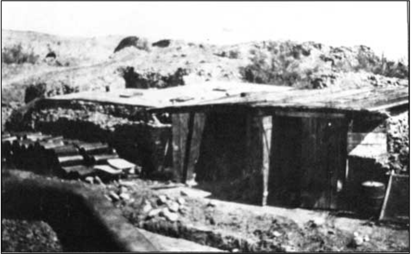
Figure 4.3. Three rooms of the southwest corner of the Aztec Ruin revamped by Morris during the 1920s for personal purposes. Unexcavated West Wing rooms are in the background.
