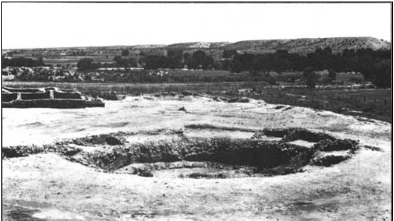
Figure 7.9. Deteriorated condition of Great Kiva prior to reconstruction in 1934.
