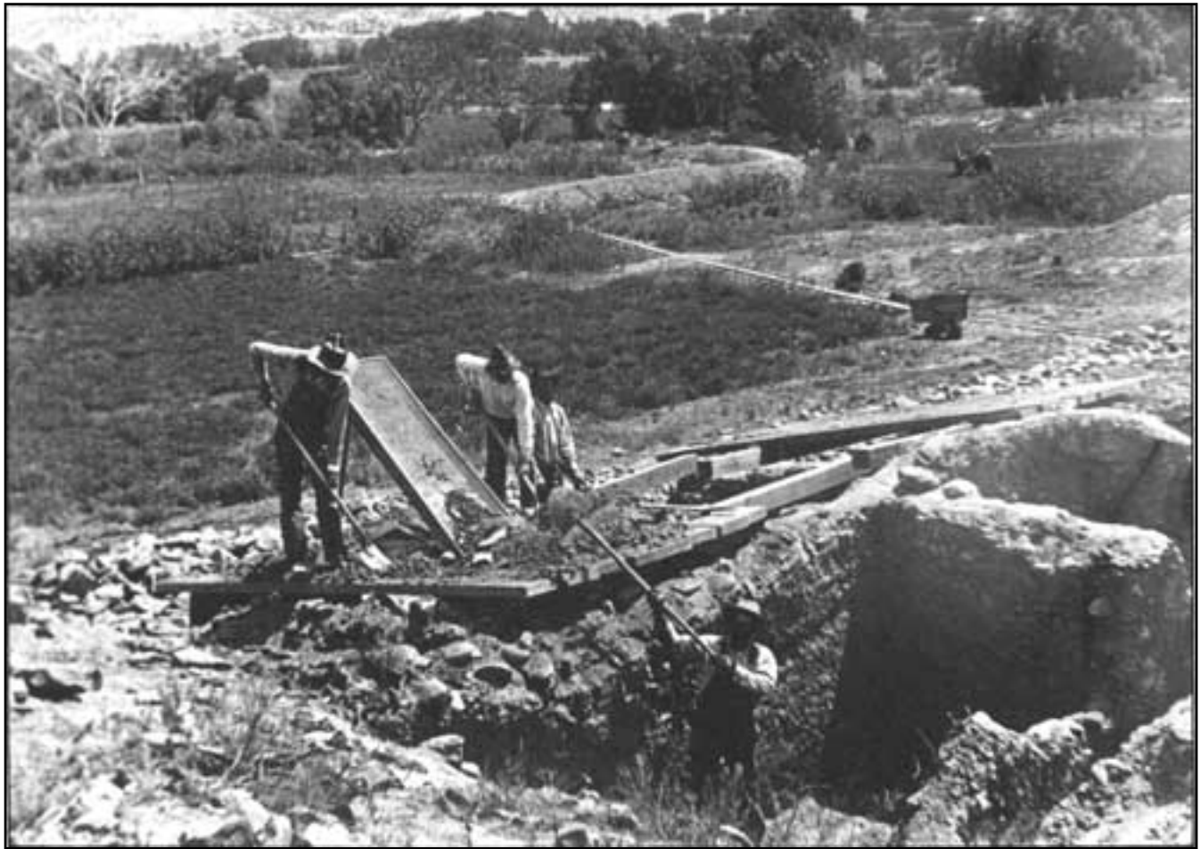
Figure 3.10. Workers in 1916 screening room fill; mine car and tracks to dump in background.
