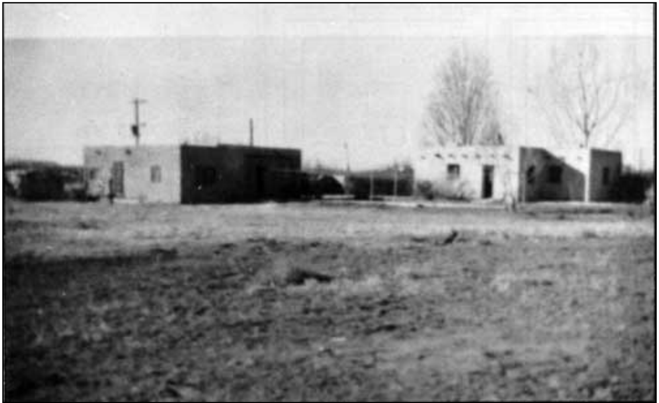
Figure 10.6. From right to left, buildings 2, 3, and 4. Photograph taken in 1949 prior to the razing of building 2.
