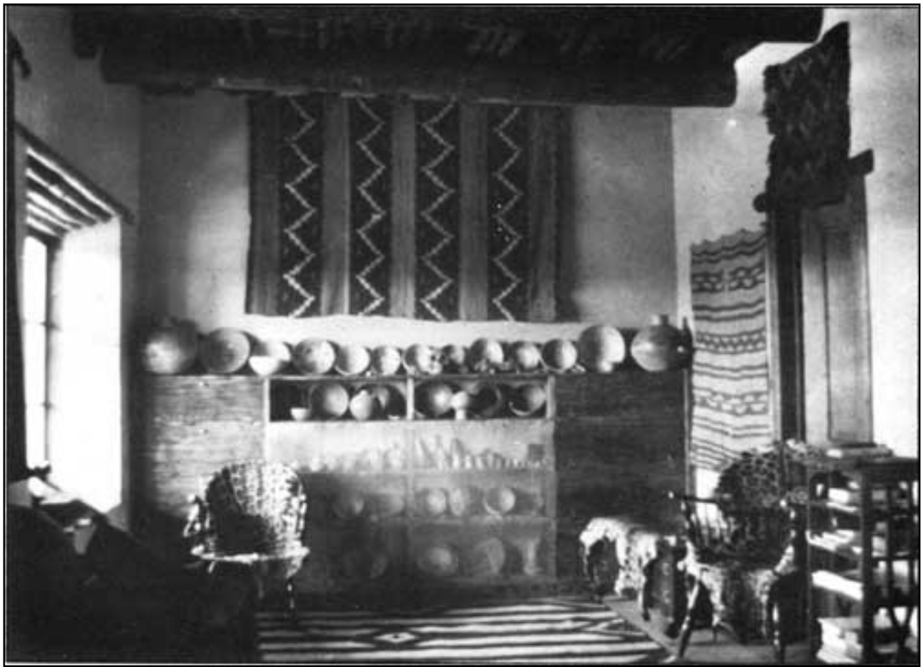
Figure 4.2. The Morris living room with collections of Indian objects. Ceiling beams are twelfth-century elements removed from the West Ruin. Window and door lintels are modern wood installed in the Anasazi way.
