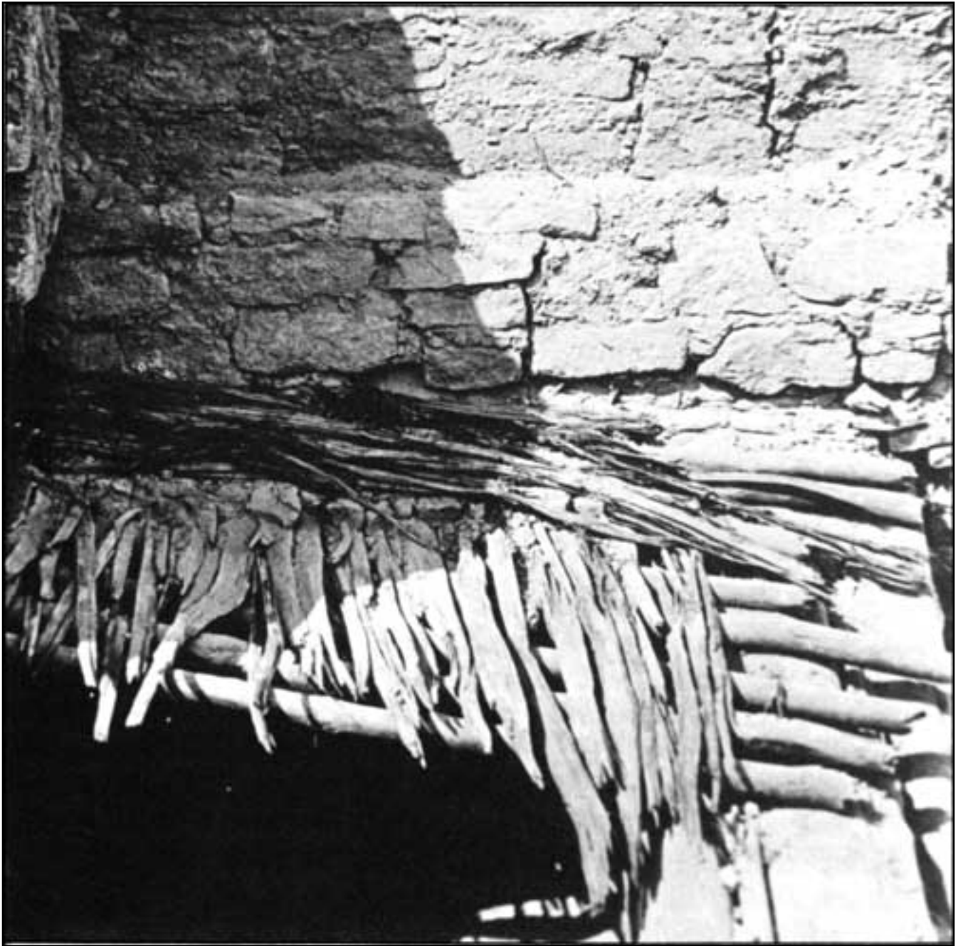
Figure 3.6. Exposed first-story roof of primary beams, cross poles, and strips of cedar bark.
