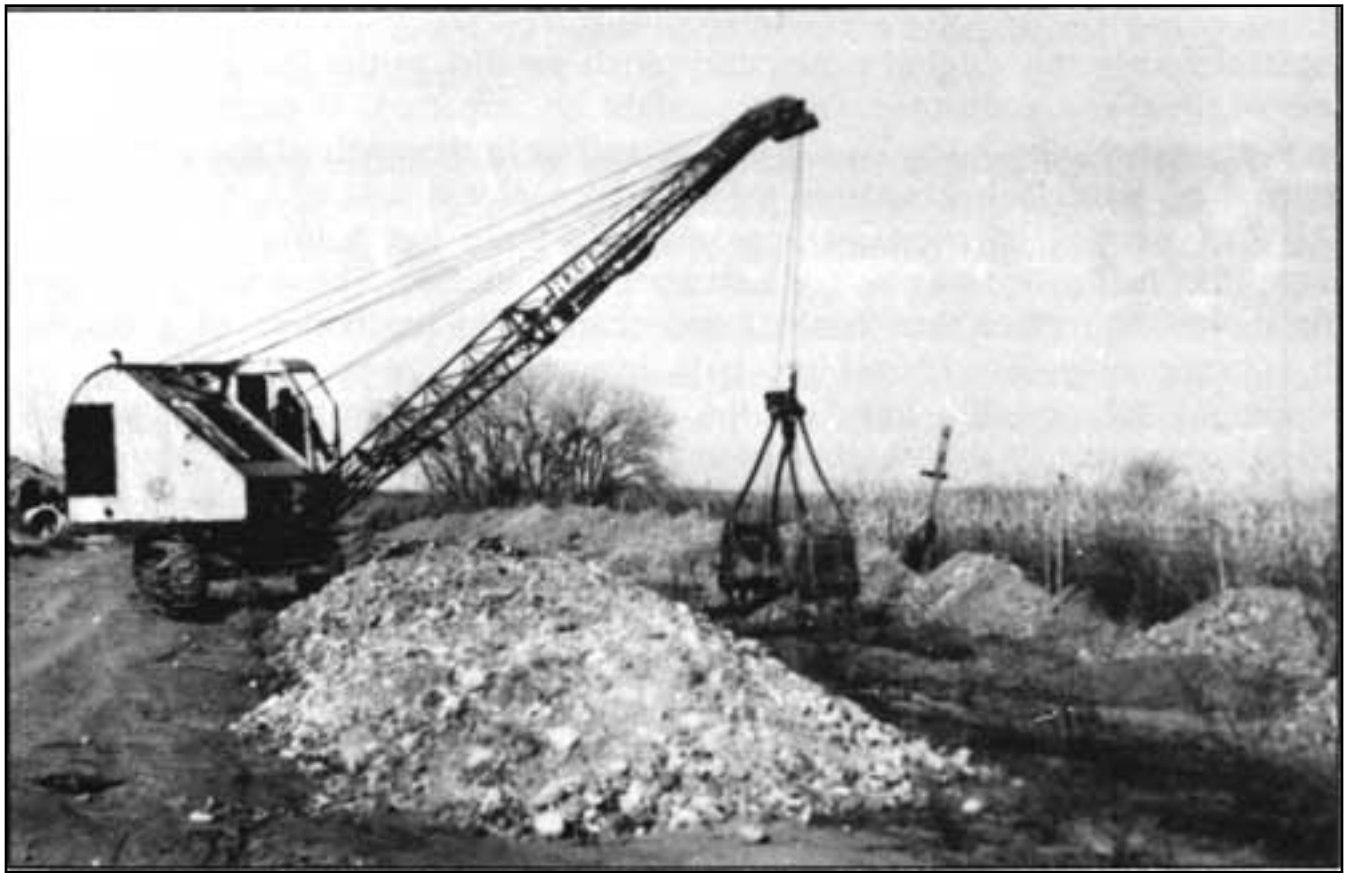
Figure 12.5. Dragline digging deep north drainage trench, 1946.
