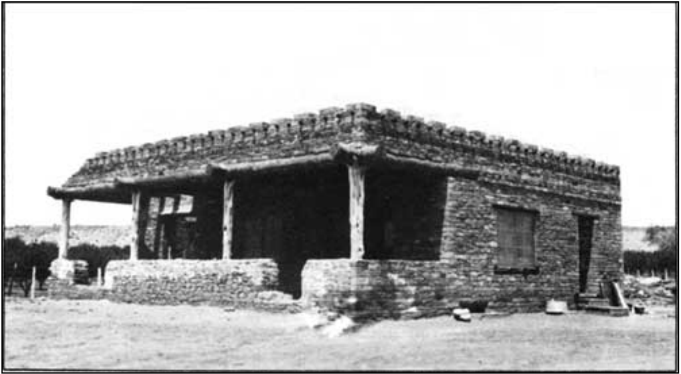
Figure 4.1. American Museum field station, built of shaped stone from Aztec Ruin and occupied by the Morris family from late 1920 to 1933, as it appeared about 1923-1924. The western room, planned as an exhibit hall, was not yet roofed.
