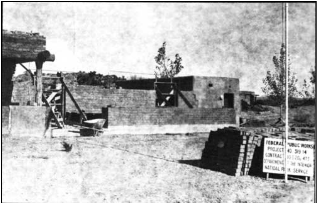
Figure 7.13. Lobby being erected between Morris house and comfort stations, 1934.
