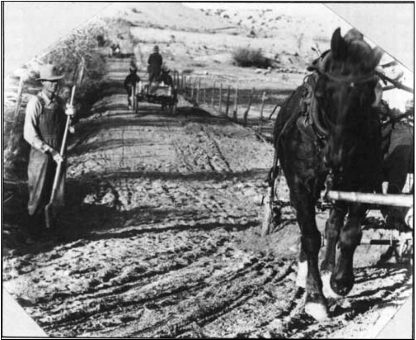
Figure 7.4. Relays of horse-drawn wagons hauling debris from West Ruin to fill ruts in entrance road, 1933.
