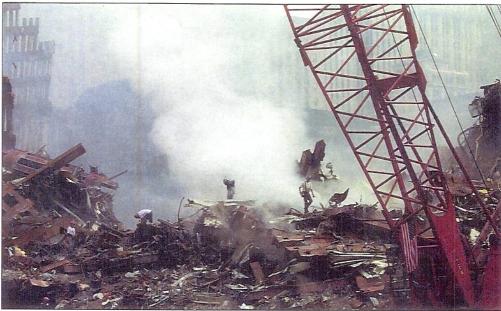
Construction workers emerging from the debris at Ground Zero.
