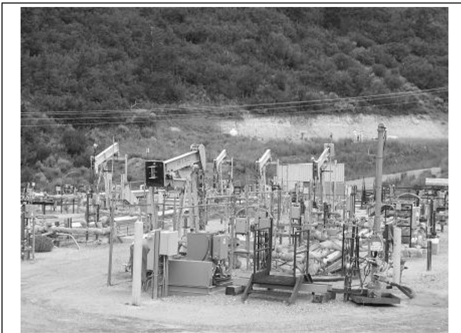
This research facility on private land in Colorado is one of several efforts underway to test techniques for oil shale development. BLM is currently preparing a Programmatic EIS which will analyze issues associated with commercial oil shale and tar sands leasing on Federal land.
