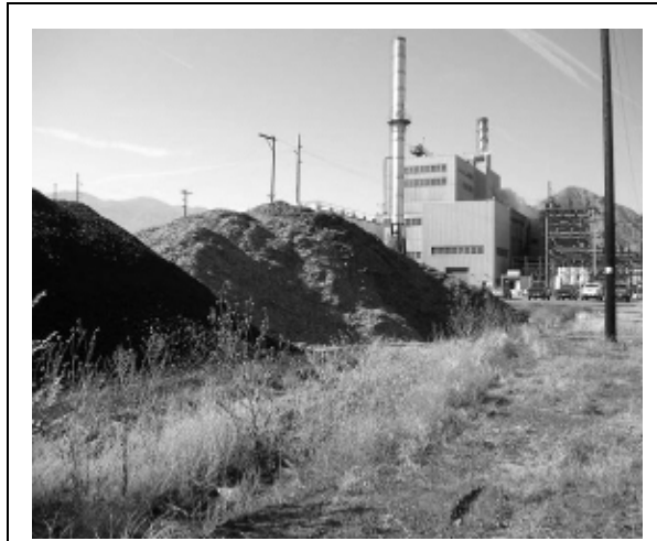
Biomass from BLM restoration treatment on the Royal Gorge Field Office in Colorado. The woody biomass is burned with coal to improve efficiency and provide renewable energy.
