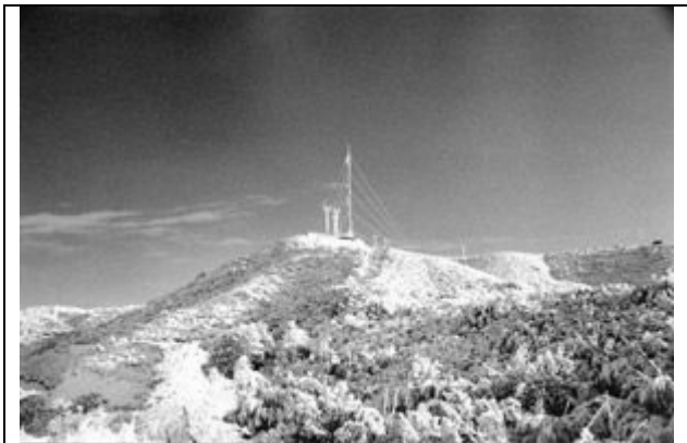
Communication site in Oregon, part of the fabric of 3,500 sites for critical modern-day infrastructure support on public lands, and 93,000 total rights-of-way.
