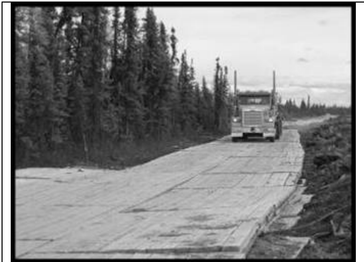
Oak pellet mats used to spread the load and reduce the imprint left on the soils and vegetation in Wyoming.
