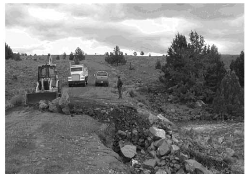
Steens Road damage repair due to floods in Eastern Oregon
