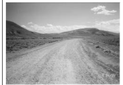
The two-track road in the upper photo is an example of a BMP used by BLM to reduce the amount of area disturbed for development and reduces visual and wildlife habitat impacts, compared with the standard road
