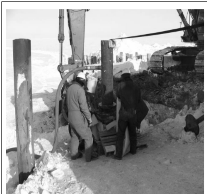
BLM uses contractors during winter months to plug legacy wells in Alaska. In this 2005 photo, crews removed thousands of gallons of diesel fuel from the J.W. Dalton well bore. The removal was necessary in order to prevent a spill, which would have damaged marine habitat in the Beaufort Sea.
