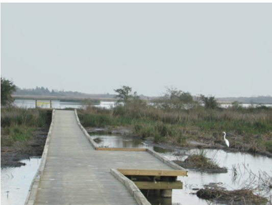
Board walk constructed over restored tidal wetlands
