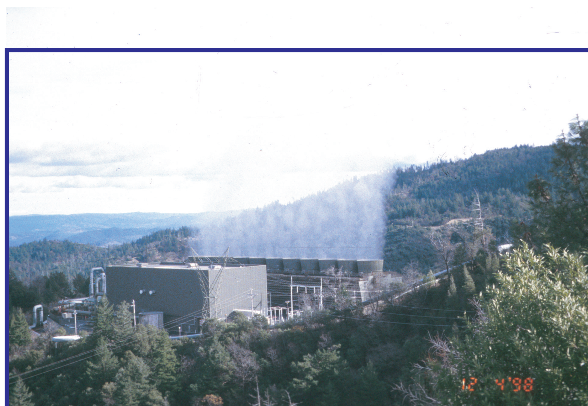
Photo looking SE of power plant (Unit 16), SE Geysers geothermal field.
