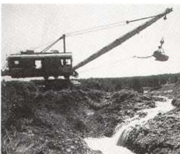
Oil-powered dredge digging a 30-foot-wide ditch to drain wetlands near Carroll, Iowa. (Photograph courtesy of National Archives, 8-D-2214-2570.)
