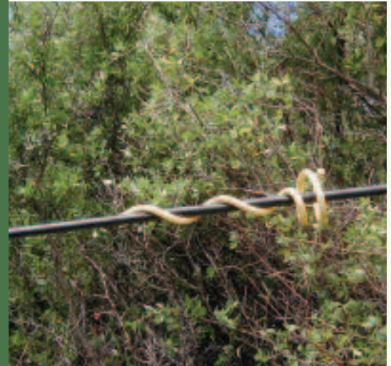
Pacific Gas and Electric Company
