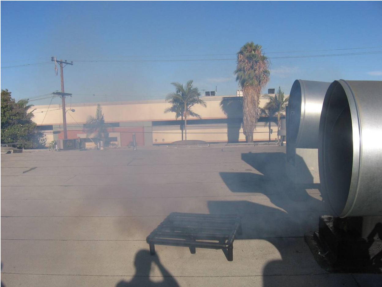
Figure 8. Rooftop re-entrainment smoke test.
