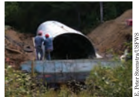
New culvert construction underway.
