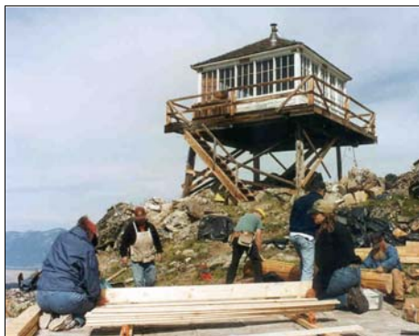
The Bitterroot National Forest in Montana used Fee Demo funds from the Recreation Lodging Program to restore the Gird Point Lookout
