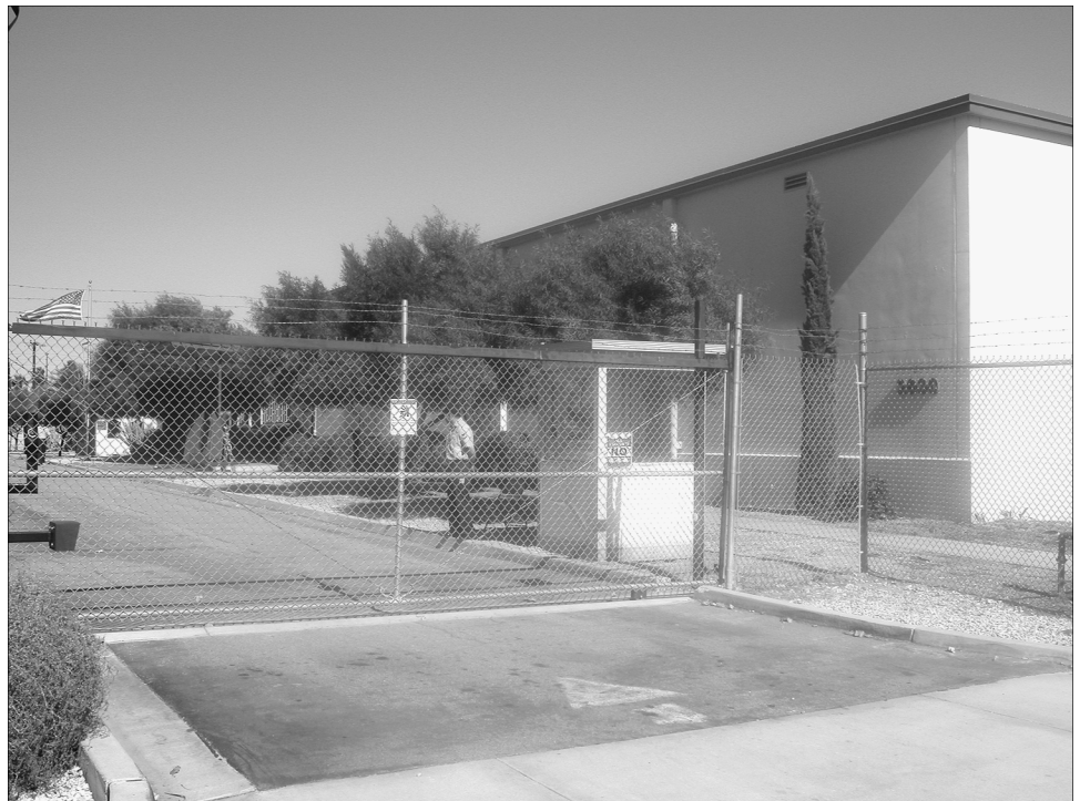
Figure 3: Navy Compound at March Air Reserve Base
