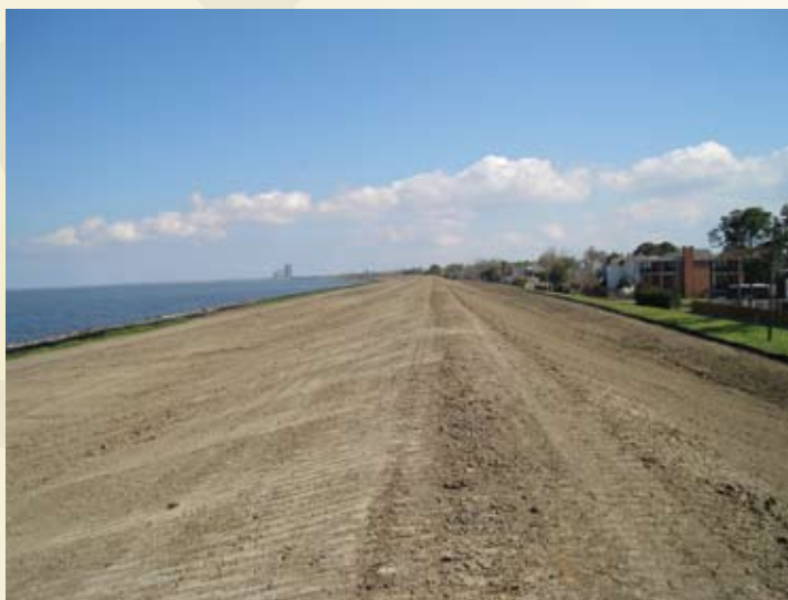
Recent upgrades that raised the height of this earthen levee increased protection against storm surge in the New Orleans area.
