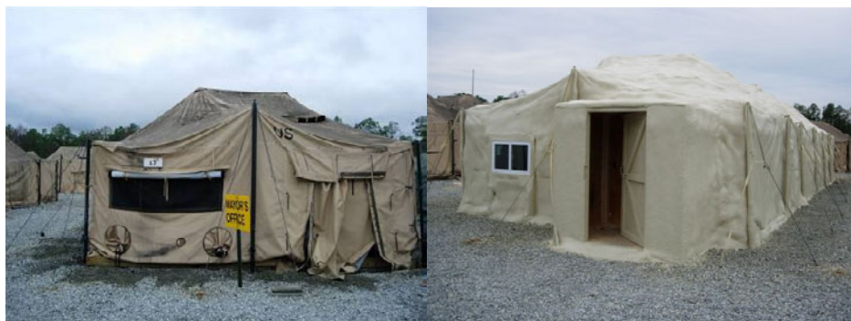
Figure: Tent before Application of Foam Insulation and Tent after Application of Foam Insulation
