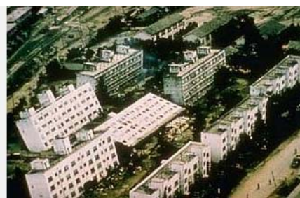
Entire buildings tilt because of ground failure after the Niigata, Japan, earthquake. Credit: NGDC.
