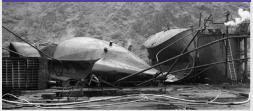
● Figure 8. WESTVACO paper mill tank failure.
