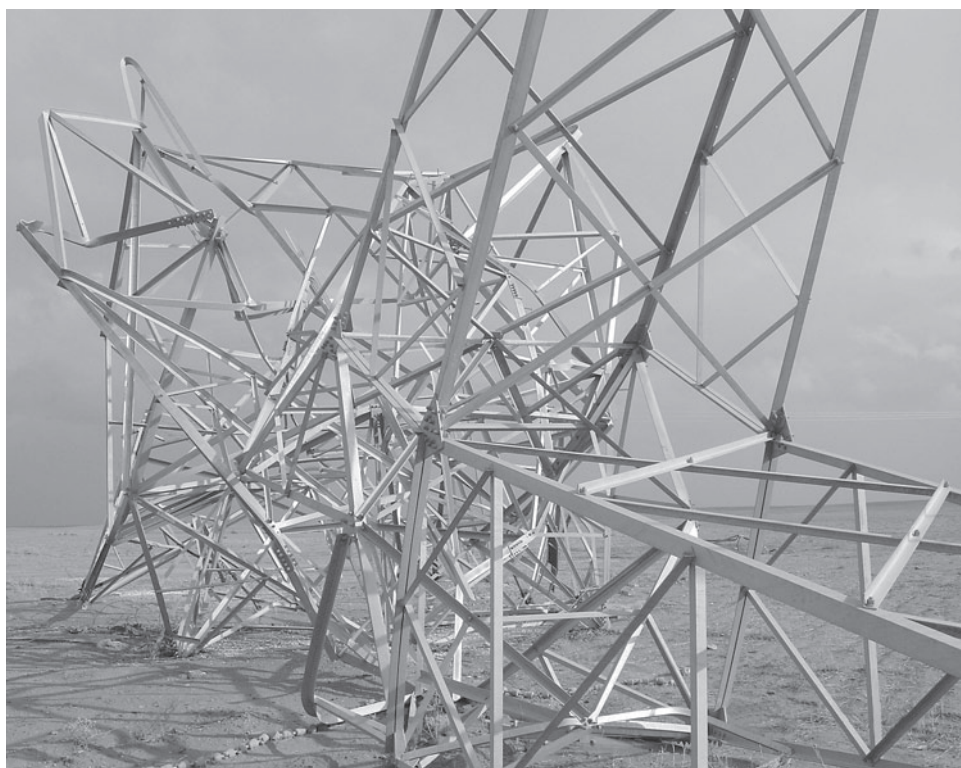
Figure 9: Downed Transmission Tower in Iraq
