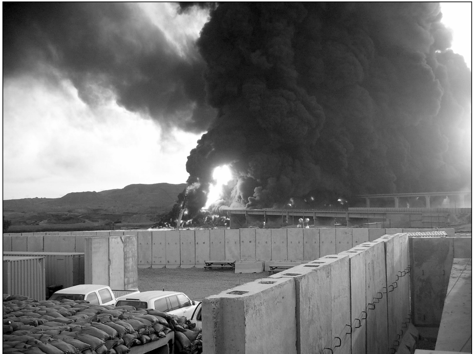
Figure 10: Attack on Oil Pipeline
