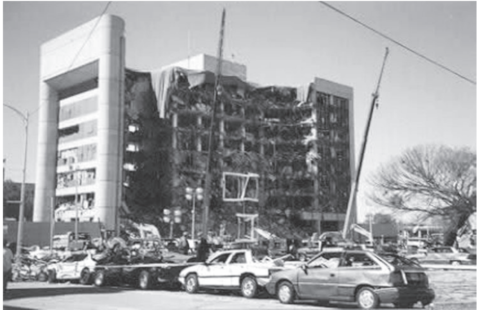
Figure 1: Murrah Federal Building, Oklahoma City
