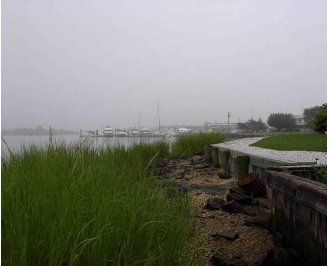
Figure 5.2 Fringing marsh and bulkhead, Monmouth County, New Jersey.
