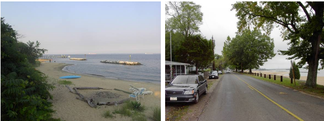
Figure 12.2 Beach nourishment along estuaries. (a) The Department of Natural Resources provided an interest-free loan to private landowners for a combined breakwater and beach nourishment project to preserve the recreational beach and protect homes in Bay Ridge, Maryland (July 2008). (b) The Virginia Beach Board and Town of Colonial Beach nourished the public beach along the Potomac River for recreation and to protect the road and homes to the left (October 2002).
