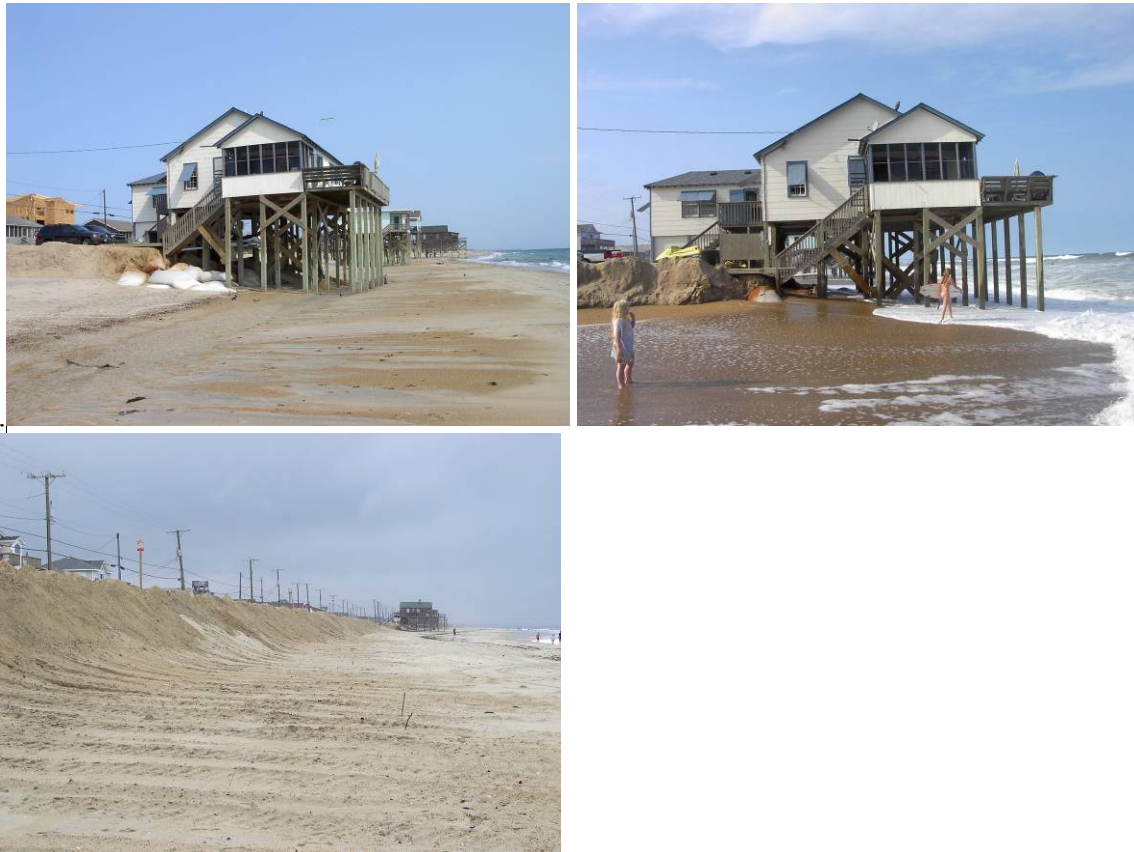
Figure 12.6 Retreat. (a) Houses along the shore in Kitty Hawk, North Carolina (June 2002). Geotextile sand bags protect the septic tank buried in the dunes. (b) October 2002. (c) June 2003
