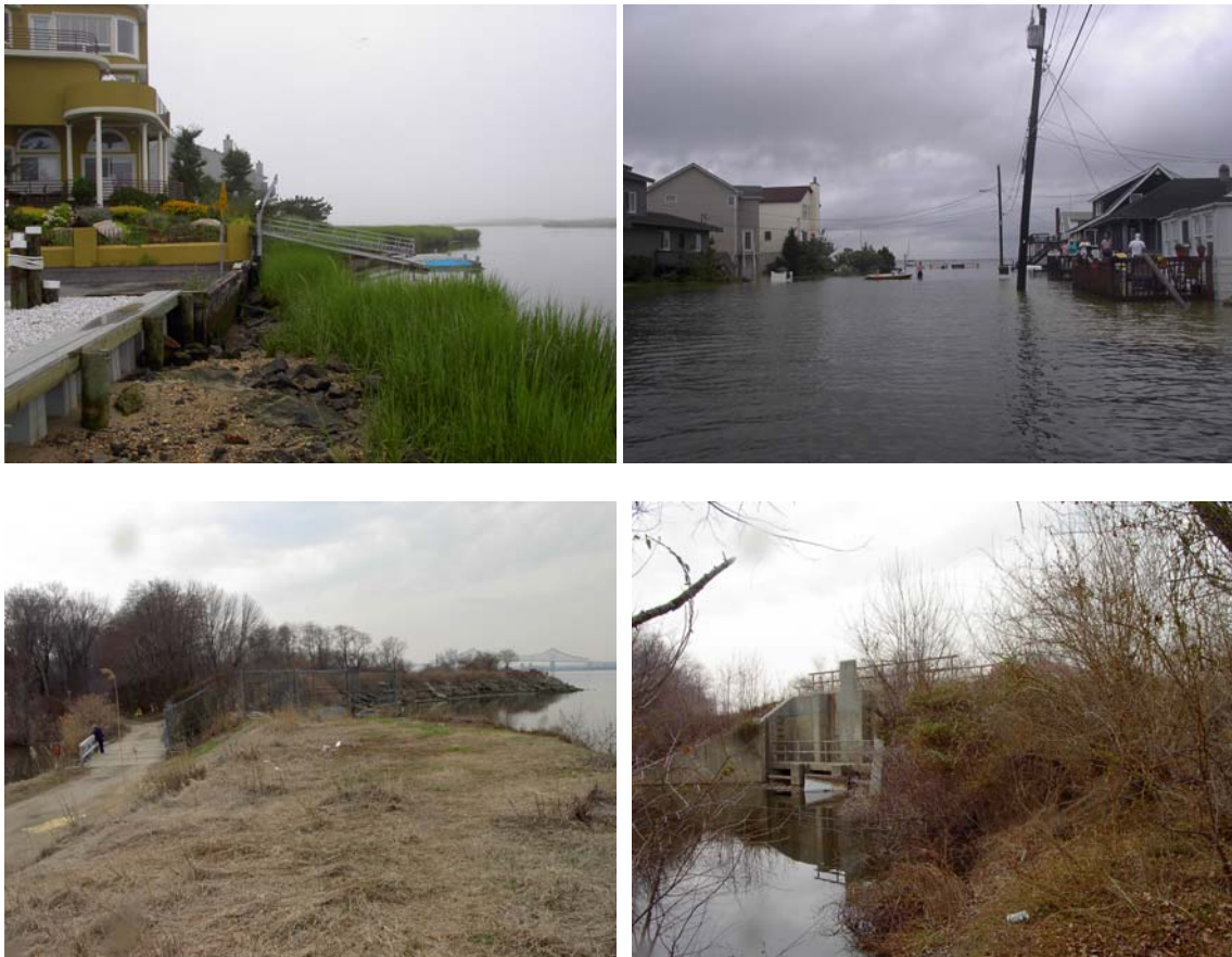
Figure 11.4 Vulnerability of New Jersey's coastal zone (a) Wetland fringe lacks room for wetland migration (Monmouth August 2003). (b) Low bay sides of barrier islands are vulnerable to even a modest storm surge. (Ship Bottom, September 2, 2006). (c) Gibbstown Levee and (d) associated tide gate protect lowlying areas of Greenwich Township (March 2003).
