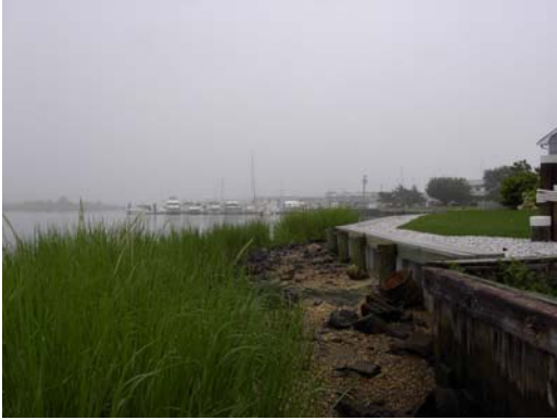
Figure 10.4 Wetland Migration thwarted by development and shore protection. Elevating the land surface with fill prevents wetlands from migrating into the back yard with a small or modest rise in sea level. The bulkhead prevents waves from eroding the land, which would otherwise provide sand and other soil materials to help enable the wetlands to accrete with rising sea level (Monmouth New Jersey, August, 2003).
