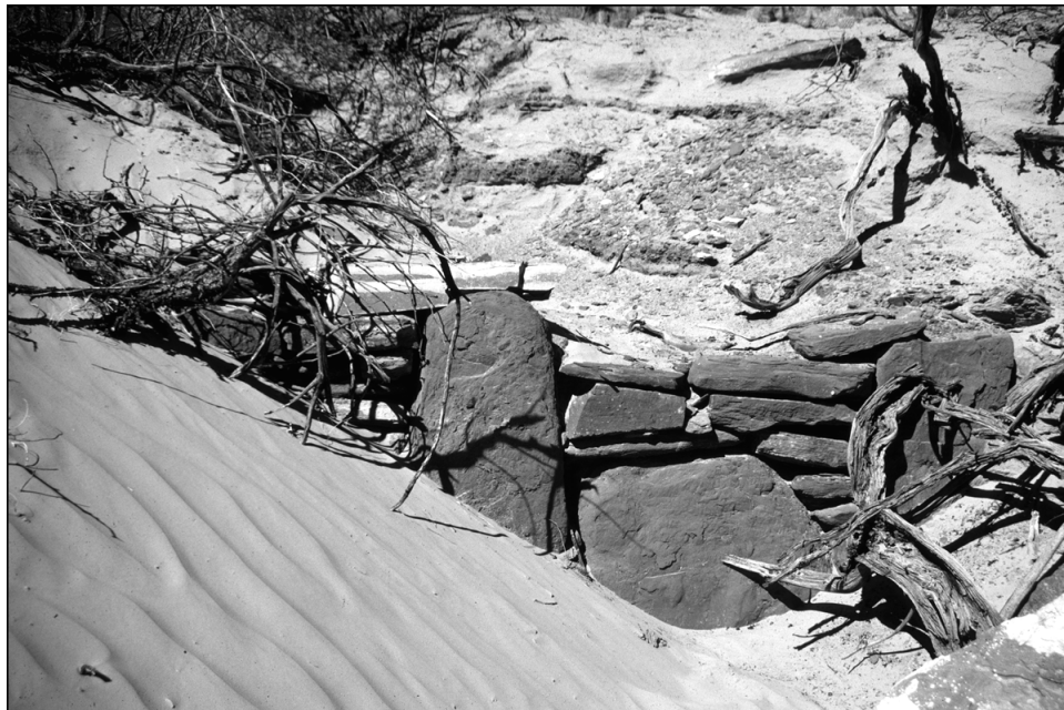
Figure 52. A Pueblo II structure at AZ C:13:10, near Unkar Delta, partially covered by drifting aeolian sand (photograph by Helen Fairley).
