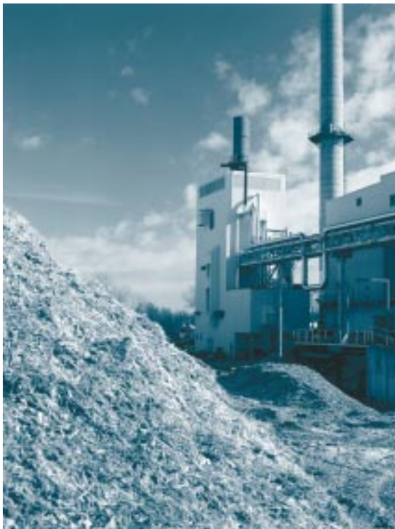
Vermont biomass gasification plant
