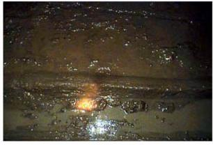
The best maintained brake car is still a hazard if the track and road bed are not maintained properly. Enough dirt, mud or debris on the rails will make the braking system ineffective. If enough dirt, mud or debris is present to slow the car's decent, a slack rope situation can develop. If the dirt or mud is allowed to accumulate on the cable rollers to the point where they won't turn, excessive wear on the cable itself can occur.
