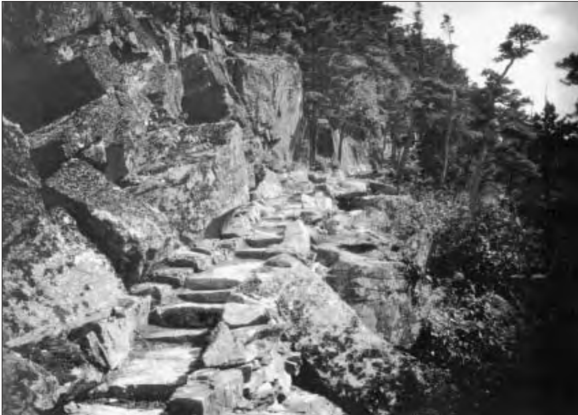
Beachcroft Path on Huguenot Head with highly crafted cut-granite steps (Acadia NP Archives).
