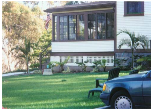
Photo 26: This is the 'Quarters A' building on FISC. The irrigated yard makes the structure appear very survivable. However, wind blown embers can get under the front porch resulting in loss of the structure. Eucalyptus trees behind these homes provide an abundance of material for ember laden winds. These non-native trees should be replaced with alternative species. A solid skirting will prevent embers from igniting the structure from below.
