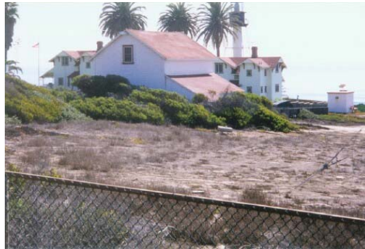
Photo 8: U.S. Coast Guard Facility on the southern tip of Point Loma. The acacia and lemonade berry growing right next to the structures will result in the total loss of the structures during a wind driven wildfire event. A minimum of 50 feet of survivable space should be maintained between the structure and the native vegetation. The acacia is an invasive exotic that spreads onto NPS lands.
