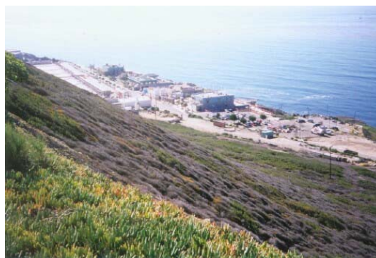
Photo 6: The Point Loma Wastewater Treatment Plant below the slope of the Western FMU.
