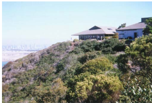
Photo 9: A view of the Cabrillo National Monument Visitor Center located above the heavily vegetated slope in the Eastern FMU.
