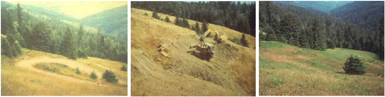
Before treatment , this abandoned logging road in Redwood National and State Parks (left photo) crossed grasslands to access timber harvest sites farther downslope. Gullies frequently form on this type of road. During road removal work , heavy equipment excavated the road bench and reshaped the hillslope to mimic natural topography (center photo). Two years following restoration work , the scar of the original road is barely visible (right photo). Note that the tree in the right foreground appears in the first photo. Photos: NPS
