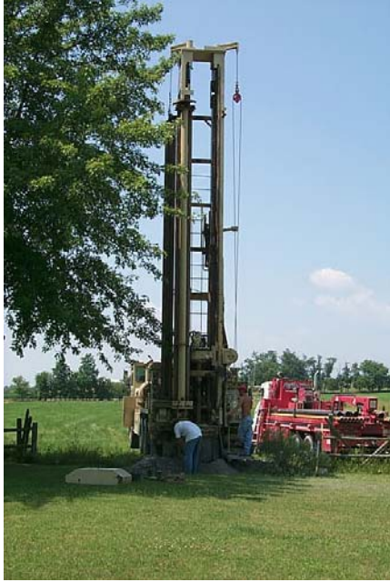
Drilling a new residential well.
