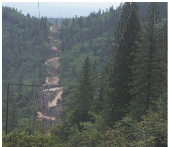
PG&E lines heading toward Old Shasta
