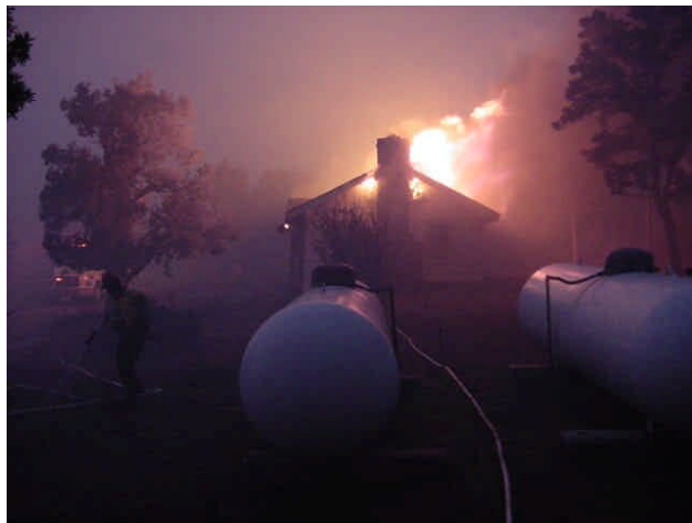
An unoccupied house is lost to embers as firefighters work to save others. The attic vent is on the other side of the house. This house also fronted a small draw coming up from the side canyon, which may have exposed it to more embers than the other structures. The hose in the center has a sprinkler between the two propane tanks.
