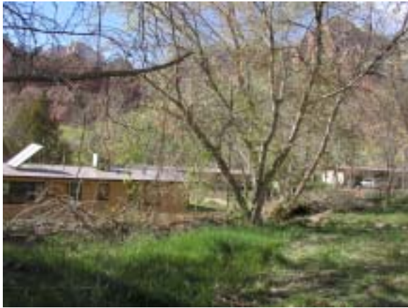
Residential area before treatment
