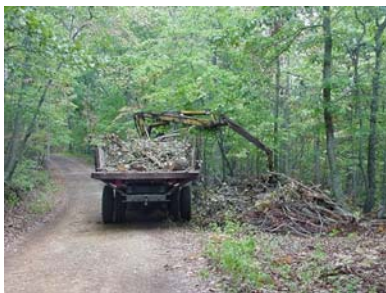
Hauling roadside piles
