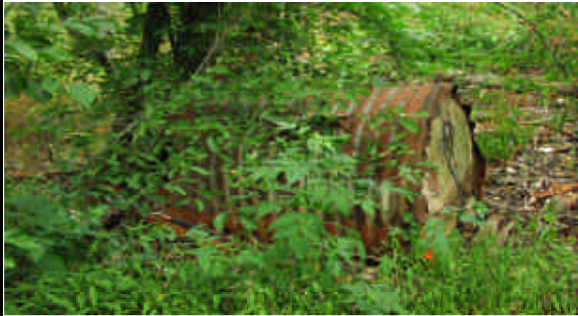
Figure 7. A section of concrete filled culvert located in Wetland 1
