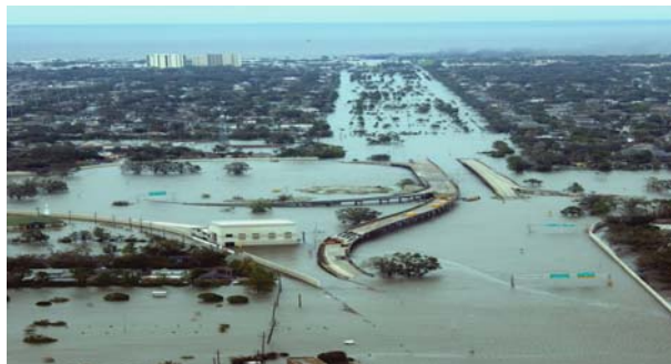
Roadways in New Orleans flooded by Hurricane Katrina. Aug. 29, 2005. Credit: Petty Officer 2nd Class Kyle Niemi, U.S. Coast Guard
