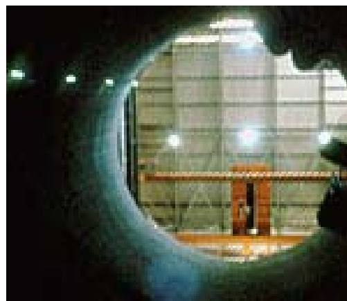
A segment of the Construction Tunnel in the LHC. Parts of the ATLAS Detector will be assembled here.
