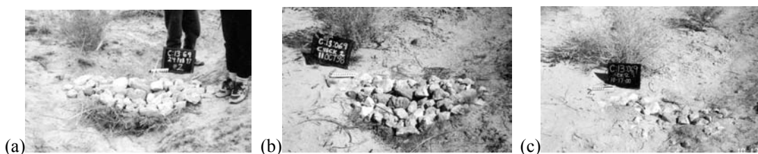
Figure 7. Site C:13:006, Checkdam 2: observed during three separate monitoring and maintenance episodes (Photo a 1997, Photo b 1998, and Photo c 2000). Note extensive sediment accumulation along both the upstream and downstream sides of the checkdam (Photo c).
