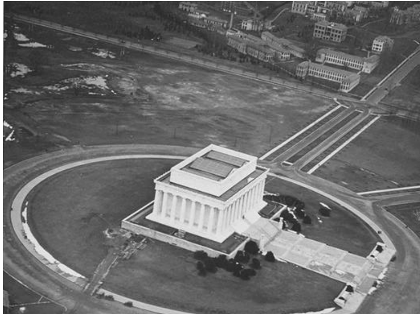
Figure 74 - Initial sidewalk installation, February 13, 1922. U.S. Navy photo. MRC 1-61.
