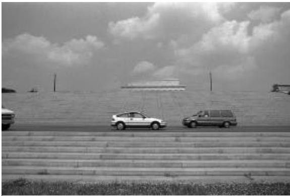
Figure 114 - Granite Watergate steps, June 1996. LINC 9-12.
