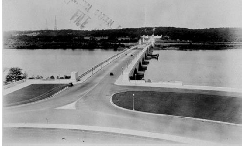
Figure 102 - Completed sidewalk and bridle trail by south plaza wing wall, June 9, 1933. MRC 1-75.
