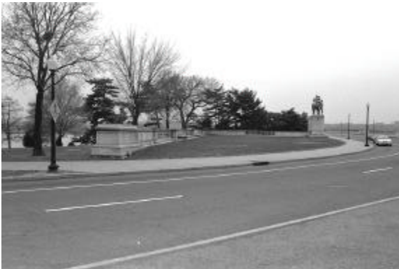
Figure 105 - South plaza wing wall with new concrete path in same alignment as original bridle path, December 5, 1996. LINC 13-1.
