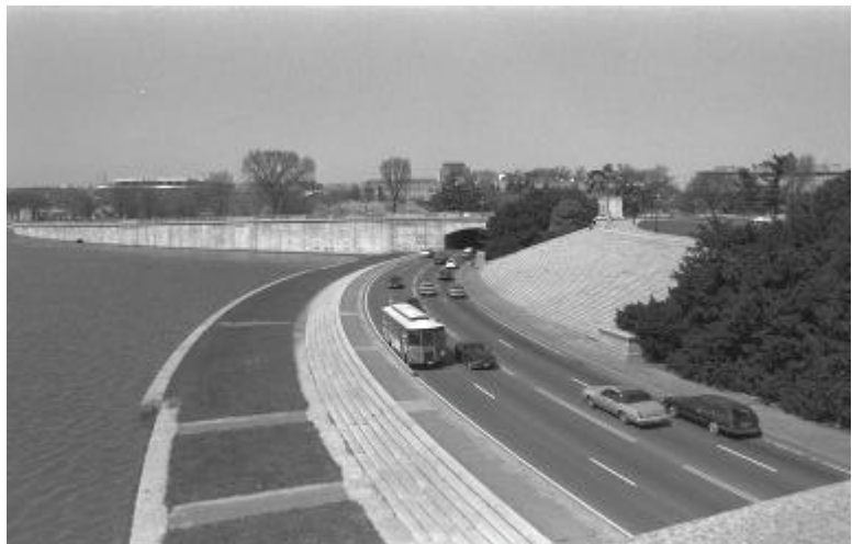
Figure 103 - Walkway on either side of Ohio Drive at base of Watergate steps, April 1996. LINC 6-15.
