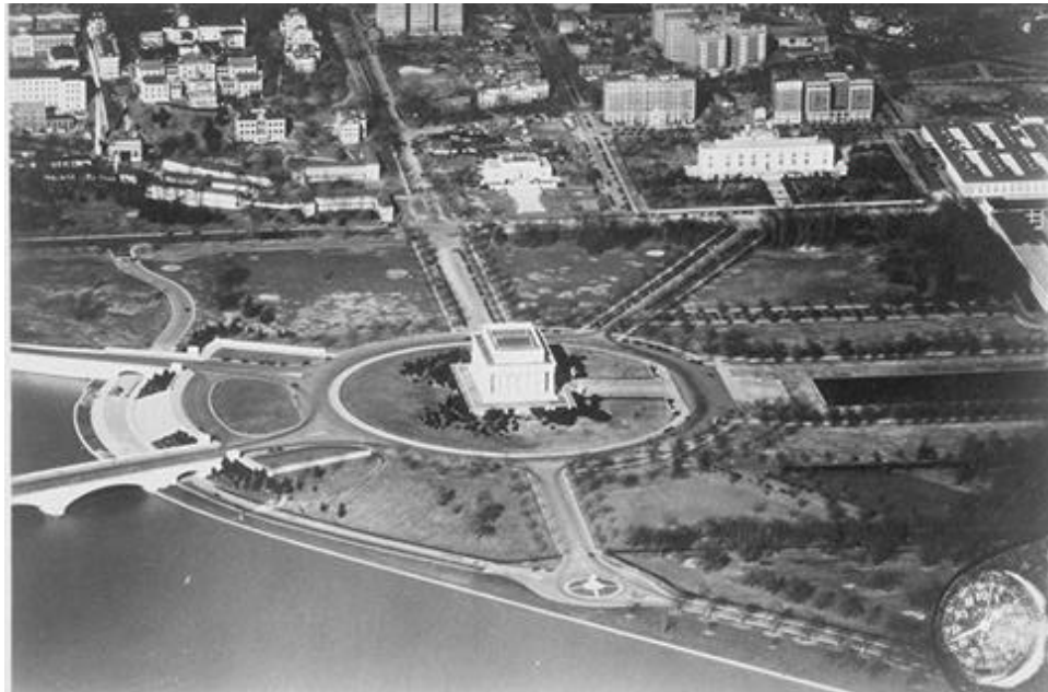
Figure 98 - Aerial view of completed road system for the Watergate area, July 1937. U.S. Navy photo. MRC I-64.
