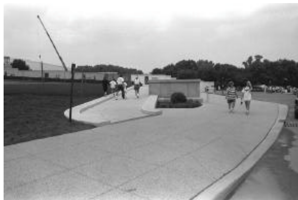
Figure 79 - Reconfigured accessible ramp to Lincoln Memorial, July 23, 1996. LINC 10-7.
