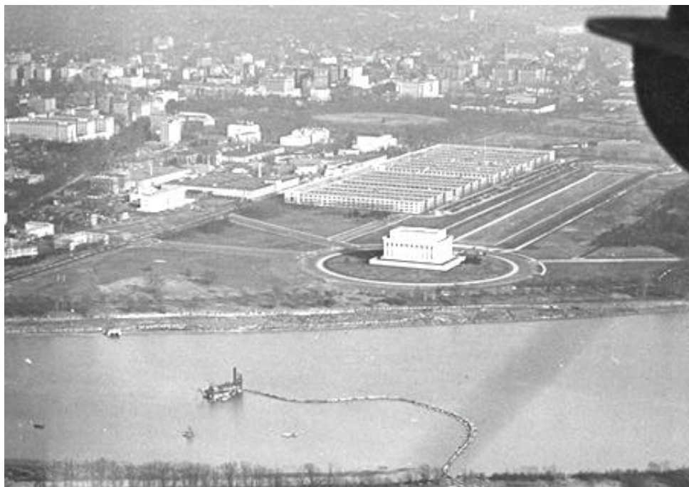
Figure 5 - Finished grading of circular road and partial completion of radial roads, 1921. MRC 1-62.
