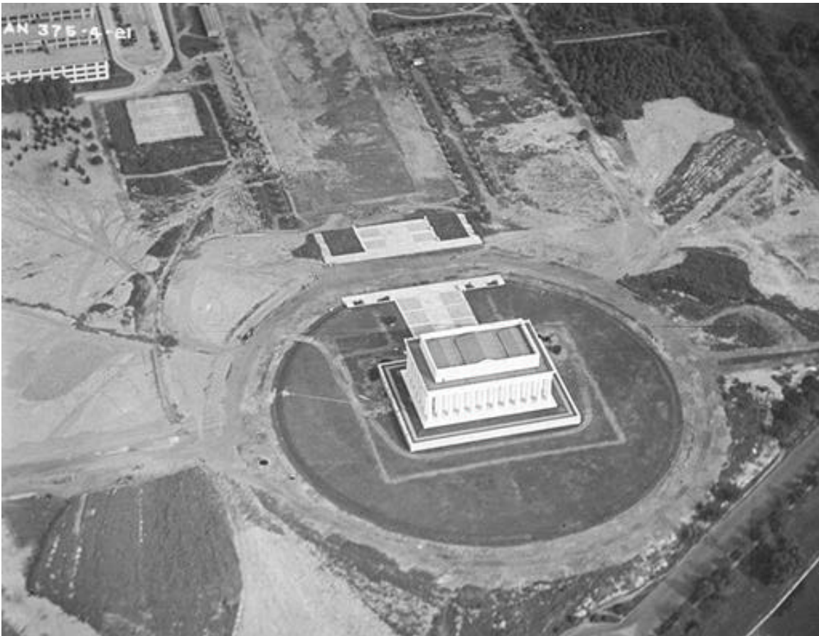
Figure 4 – Grading operations around the memorial, April 17, 1921. MRC 1-60.
