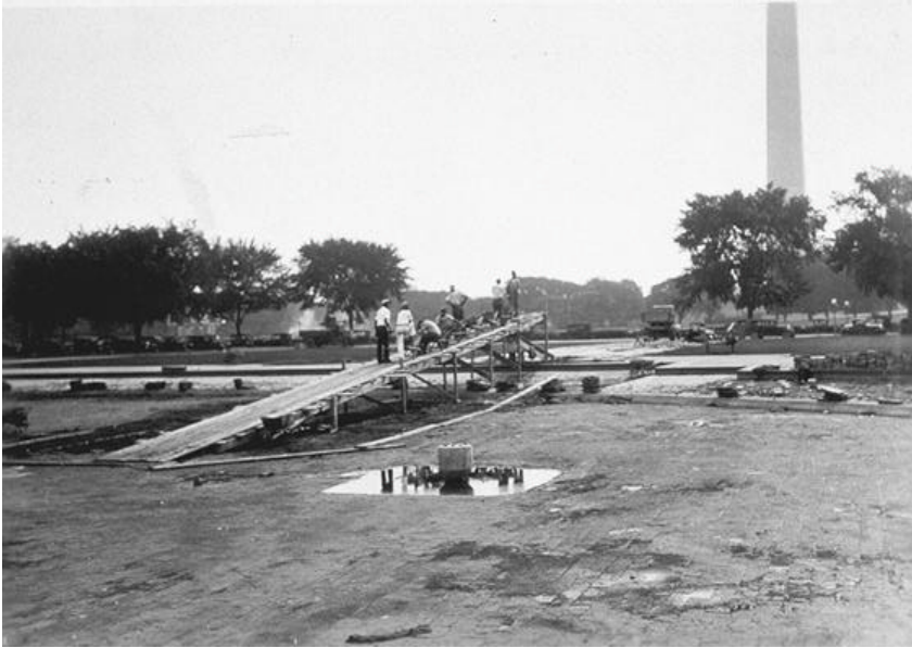
Figure 18 – Repair work to the Rainbow Pool, July 15, 1929. MRC 3-17.
