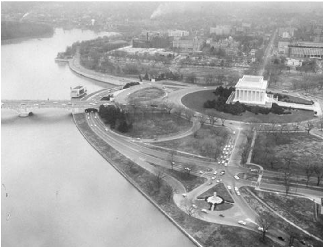
Figure 25 - New configuration of road system, with the addition of Independence Avenue and the on and off ramps from Lincoln Circle, January 27, 1960. MRC 1-108.
