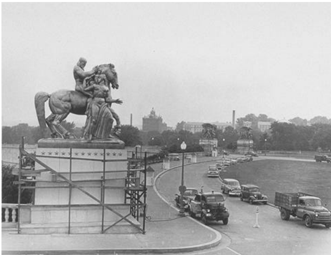
Figure 27 - Installation of "Sacrifice" statue on north side of entrance to Arlington Memorial Bridge, June 1951. MRC 1-76.
