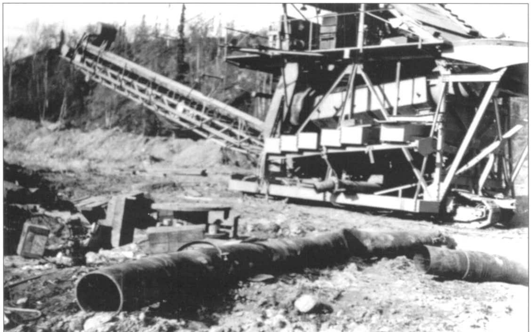
The Carrington Company’s introduction of large-scale, mechanized mining technology in 1939 brought an end to small-scale mining methods on Caribou Creek. The dryland dredge, shown above in 1939, was operated until 1942. Alaska Road Commission Collection, 61-18-138, Alaska State Library
