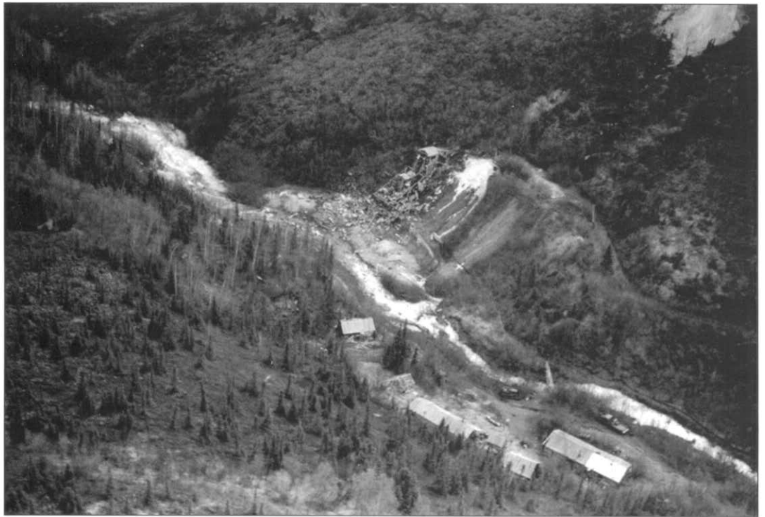
This view of the Stampede Mine mill and lower camp was taken on May 19, 1987, shortly after the April 30 explosion that demolished the mill and the nearby assay building, and seriously impacted other structures at the site. Resource Management Slide File, NPS
