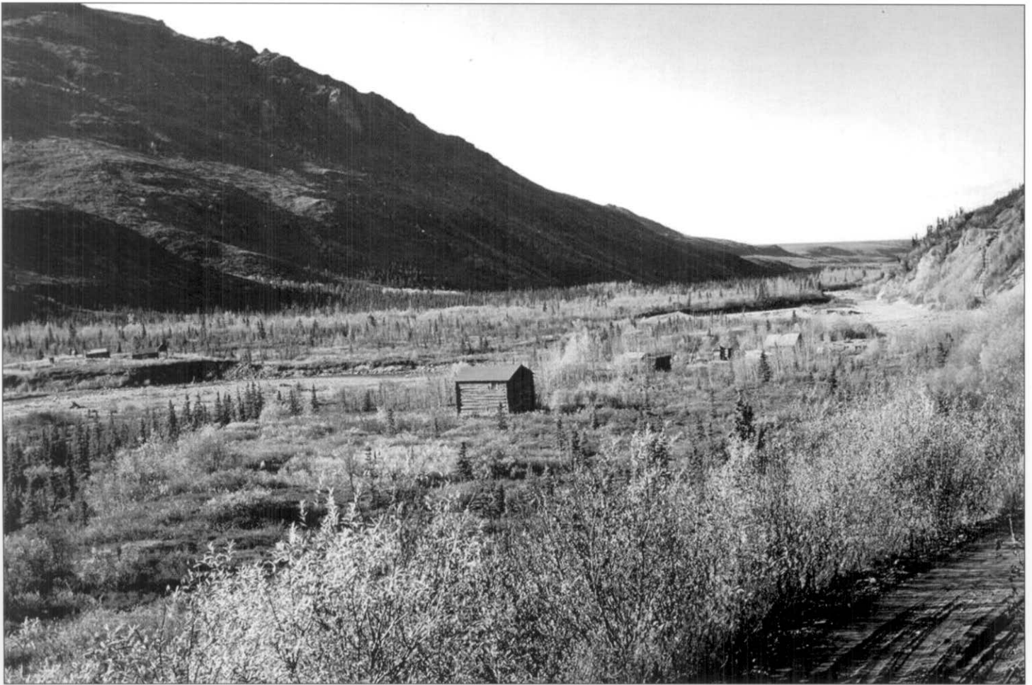
By the time this photograph was taken in 1956, only a handful of permanent residents lived in the Kantishna area. Abandoned cabins were often “recycled” for new construction or firewood in this area where timber was hard to get. The two-story Kantishna Roadhouse, center, and the Busia cabin, left, are still standing in 2008. Charlie Ott Photo, Denali National Park and Preserve Museum Collection
