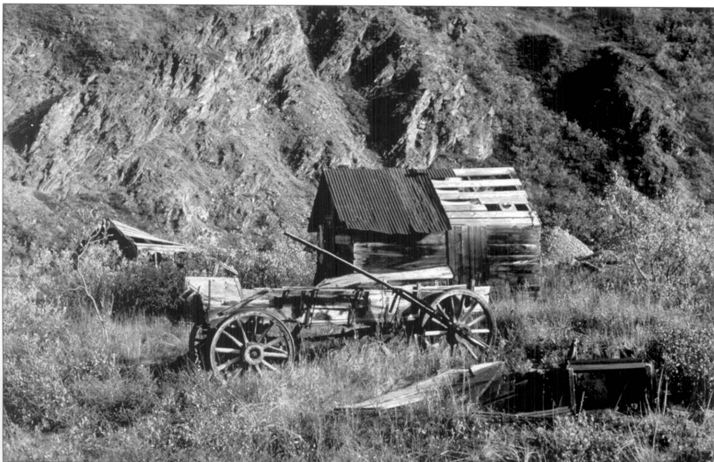
Located on upper Caribou Creek, the remains of a wooden tool shed and a wooden freight wagon (pictured above in 1984) represent historic mining activities including transportation, habitation, maintenance, mining, and mineral processing during the Carrington Company's operations from 1939 to 1948. Claire Roberts Photo, NPS, WAGS Collection
