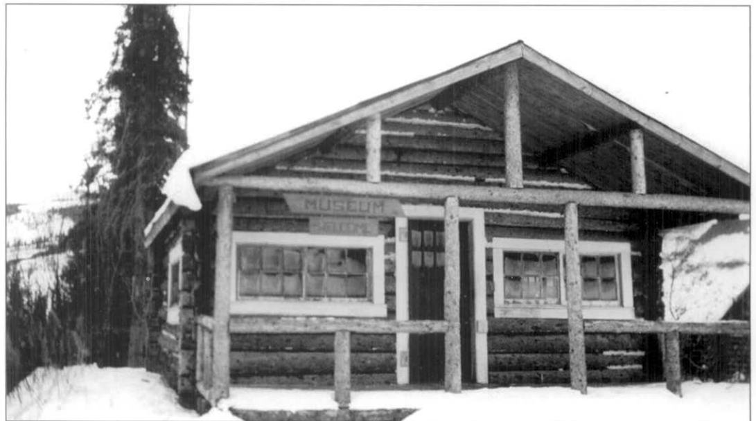
Constructed in 1926, the original Superintendent’s Office at park headquarters served as the administrative office until mid-1941, when the one-room building was considered “dilapidated.” By the spring of 1943 the building, still in its original location, was adapted for reuse as the park’s first museum. DENA 4-2.7, Denali National Park and Preserve Museum Collection
