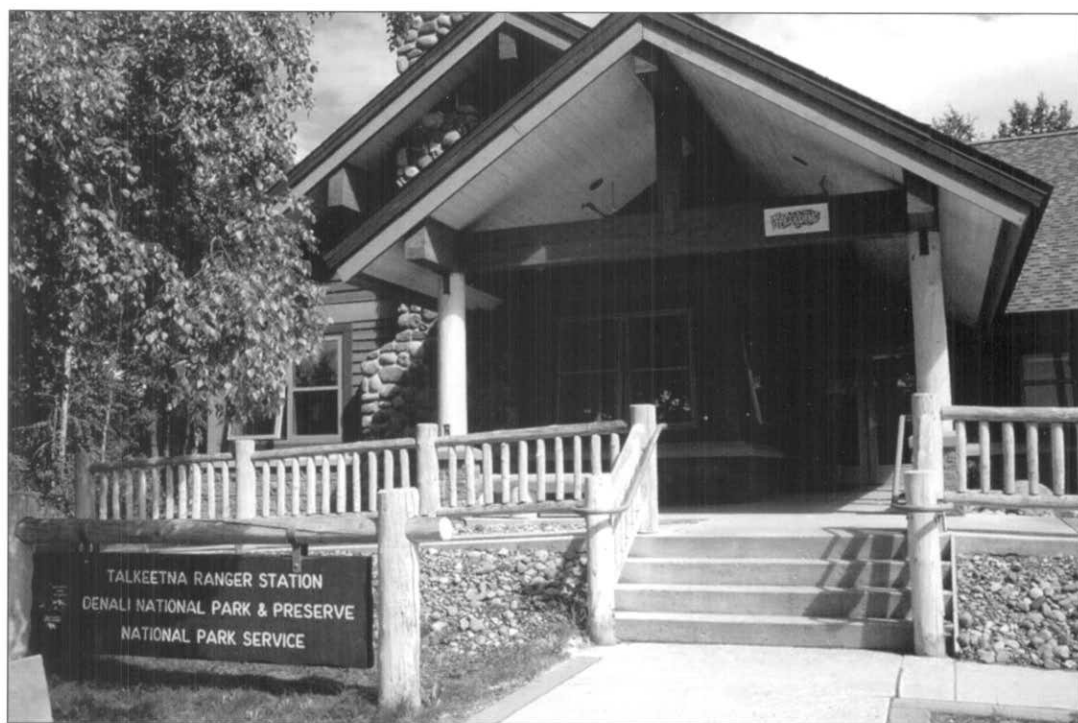
The new Talkeetna Ranger Station opened in the spring of 1997. It provides offices for the Talkeetna NPS staff, areas for mountaineer orientation and visitor contacts, and a base for search and rescue operations. NPS Photo
