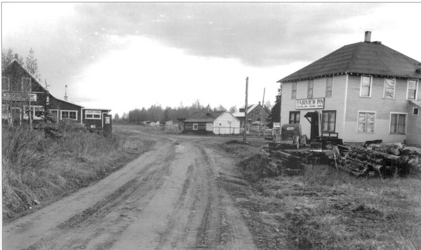
The town of Talkeetna became the hub for mountaineering access to Mt. McKinley by airplane. The airport was a small village strip adjacent to the town, and can be seen at the end of the road in this 1956 photo, which looks south. Alaska Railroad Collection, BL79-2-3857, Anchorage Museum of History & Art
