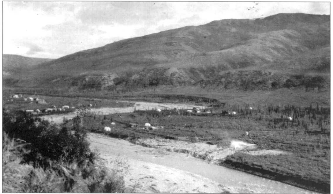
The first large-scale hydraulic operation on Moose Creek was conducted by the Kantishna Hydraulic Mining Company. This photo, looking upstream, was taken on July 10, 1922. Steel pipe brought water from the ditch to the hydraulic mining site (in foreground, on far side of Moose Creek). P.S. Smith, 1404, U.S. Geological Survey
