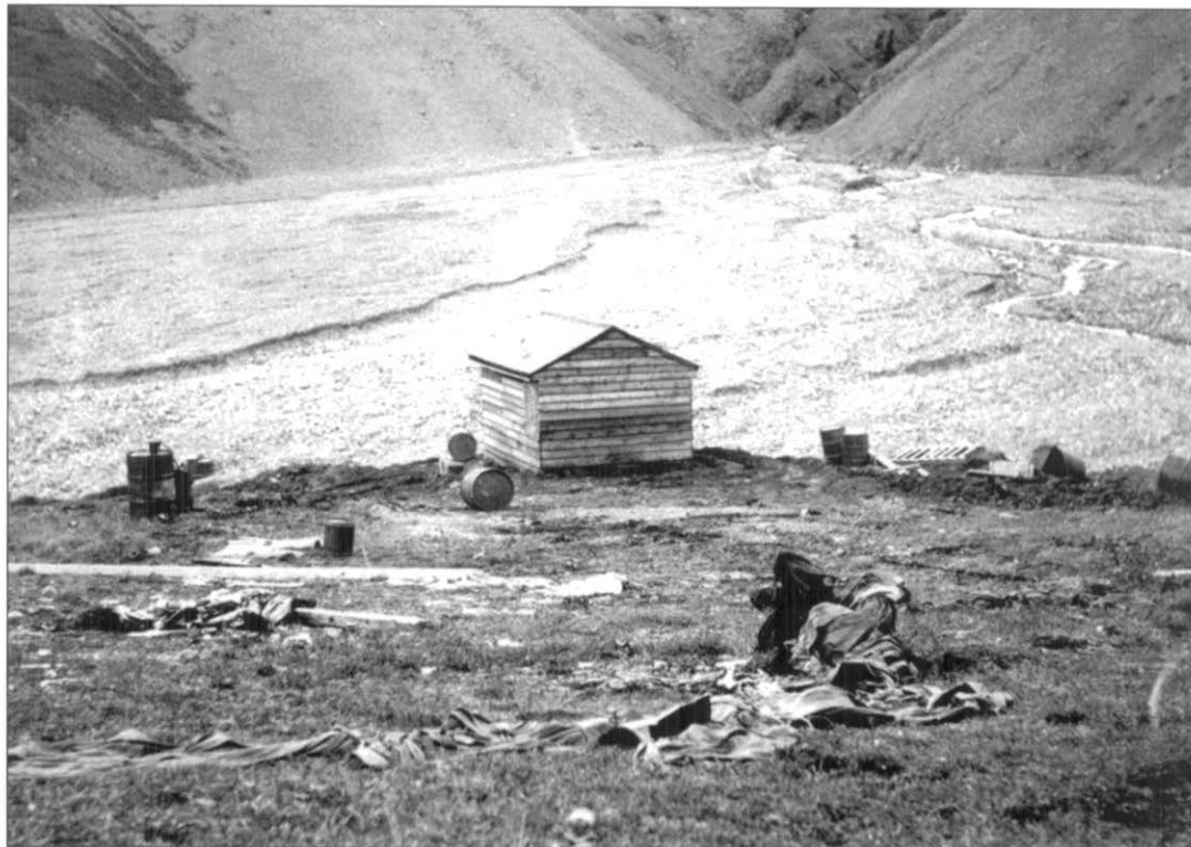
In 1963, remains of the abandoned limestone claim on the West Fork of Windy Creek included this small frame building, bulldozer cuts, oil barrels, an eroding landing strip, and a "cat trail" connecting the claim to the railroad. DENA 16-37, Denali National Park and Preserve Museum Collection
