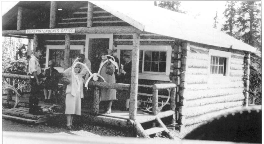
As this July 1, 1927 photo shows, park visitors stopped by the superintendent's office at park headquarters on their way from the railroad station to their destination at Savage Camp. Haskell Photo, DENA #14976, Denali National Park and Preserve Museum Collection
