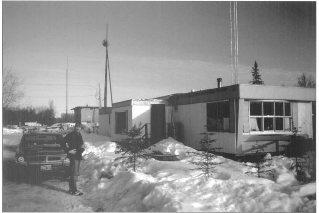
The first NPS ranger residence in Talkeetna was this mobile home, located just west of the railroad tracks. Roger Robinson Photo
