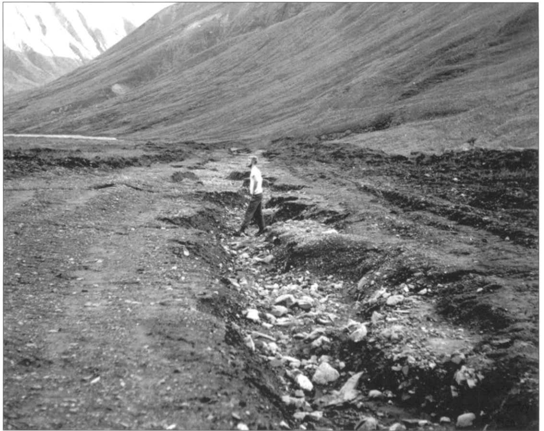
By September 1963, when this photo was taken, the 7-year-old landing strip on the West Fork of Windy Creek (which was adjacent to a potential limestone development area) had suffered considerable erosion. DENA 16-33, Denali National Park and Preserve Museum Collection
