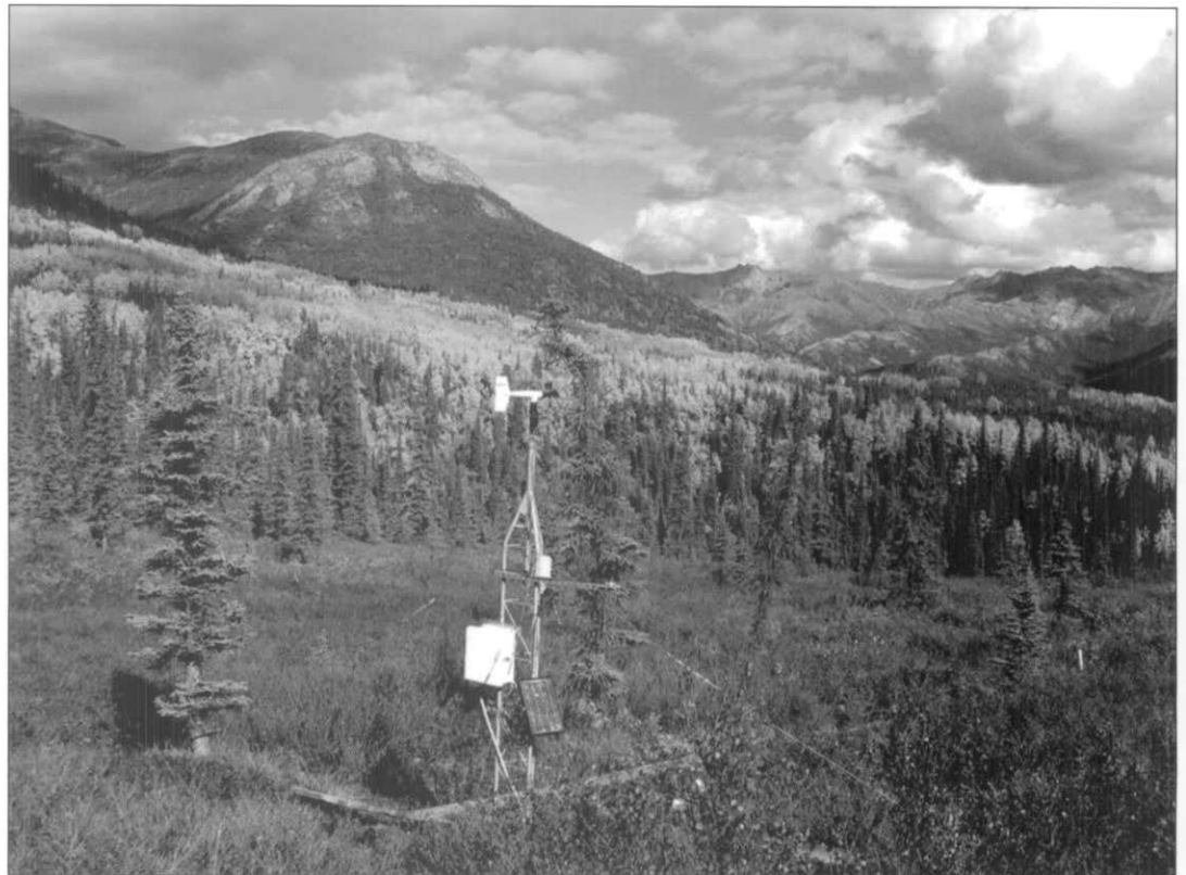
The Permafrost weather station is one of five Long-term Ecological Monitoring (LTEM) weather stations installed in 1994 to record long-term variations in climate at different elevations. The station, which is powered by a deep-cycle battery and charged with a solar panel, measures and records air temperature, relative humidity, wind speed and direction, and solar radiation. The site is located in the Rock Creek drainage adjacent to park headquarters where water and air quality, vegetation, and small mammals are also monitored as part of the Central Alaska Inventory & Monitoring Network. NPS Photo
