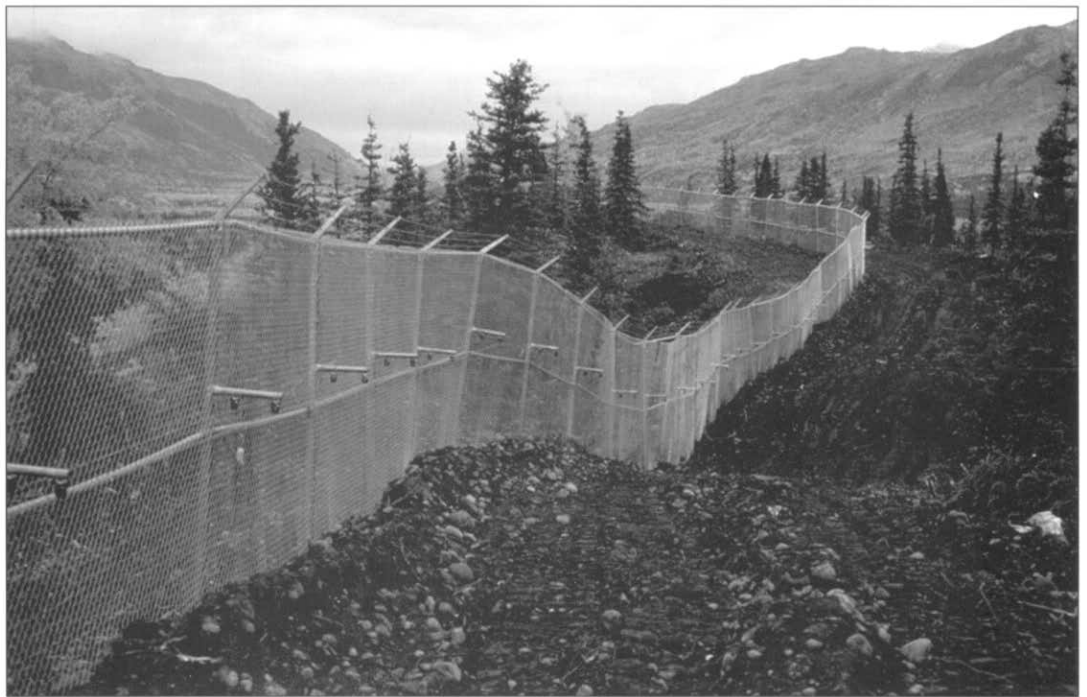
By 1975 this electric fence prevented bears from obtaining human food at the park garbage dump. Chip Downing Photo, NPS Photo, Denali National Park and Preserve
