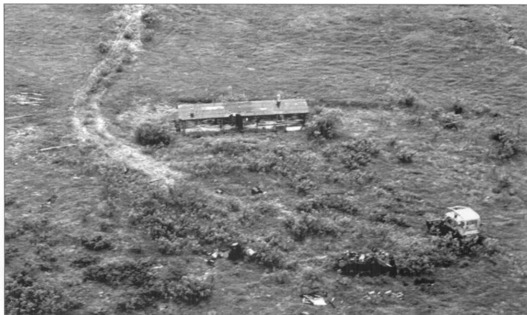
The two Caterpillar tractors that were driven from Wonder Lake to Slippery Creek mine in 1969 are pictured here at the Slippery Creek cabin in 2007. This equipment was utilized for production at the antimony mine at least through the 1975 season. NPS Photo
