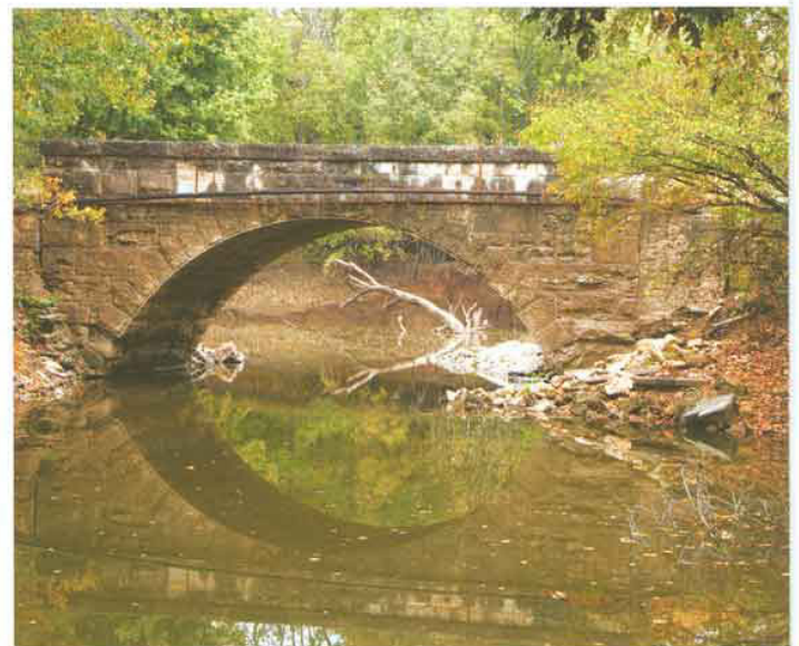
Fox Creek Bridge
