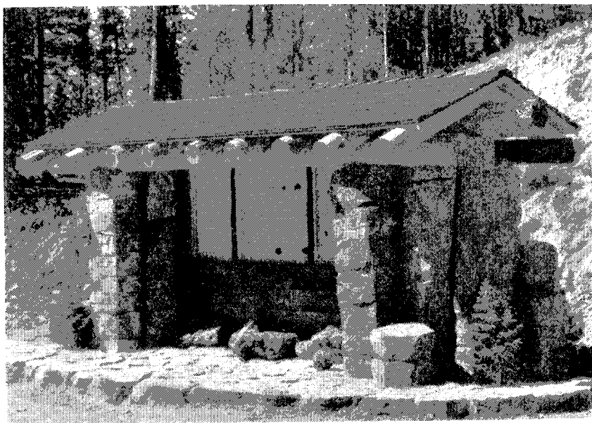
Figure 39. —TRAILSIDE EXHIBIT, OBSIDIAN CLIFF, YELLOWSTONE NATIONAL PARK, WYOMING. NOTE LARGE SPECIMENS ON FLOOR AND COMPOSING SUPPORTS OF STRUCTURE
