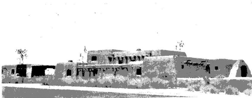
Figure 4. —MUSEUM AND ADMINISTRATION BUILDING, WHITE SANDS NATIONAL MONUMENT, NEW MEXICO
